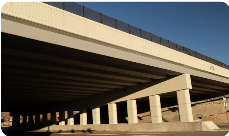
Image 20 & 21. New I-70 ML over W. 32nd Avenue Structures
