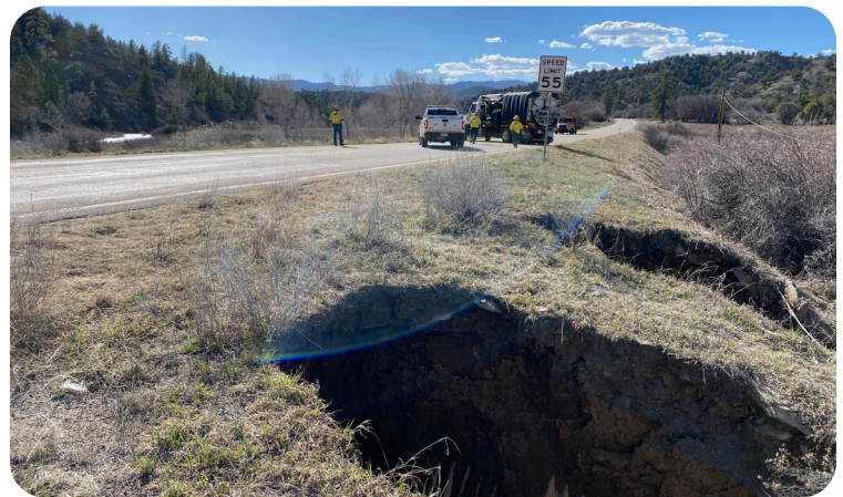
Image 8 & 9. Erosion and Settlement Around the Original Structure SH 151 ML over Stollsteimer Creek (P-07-S)
