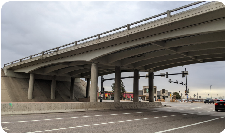
Image 16. Original I-70 ML over W. 32nd Ave Structure
