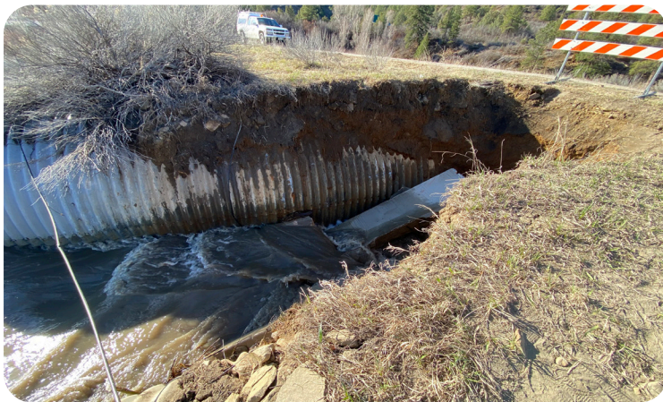
Image 8 & 9. Erosion and Settlement Around the Original Structure SH 151 ML over Stollsteimer Creek (P-07-S)
