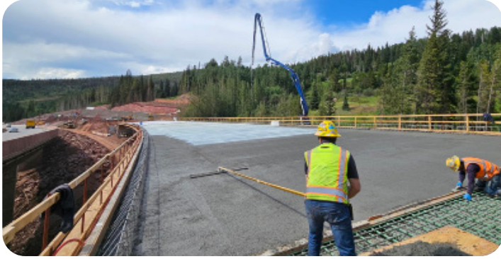
Image 24. New Bridge Deck of the future I-70 WB over Polk Creek
