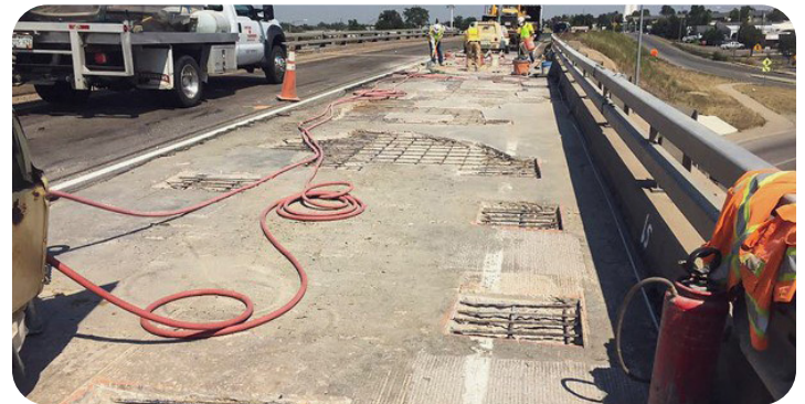
Image 25. Emergency Repairs on I-270
