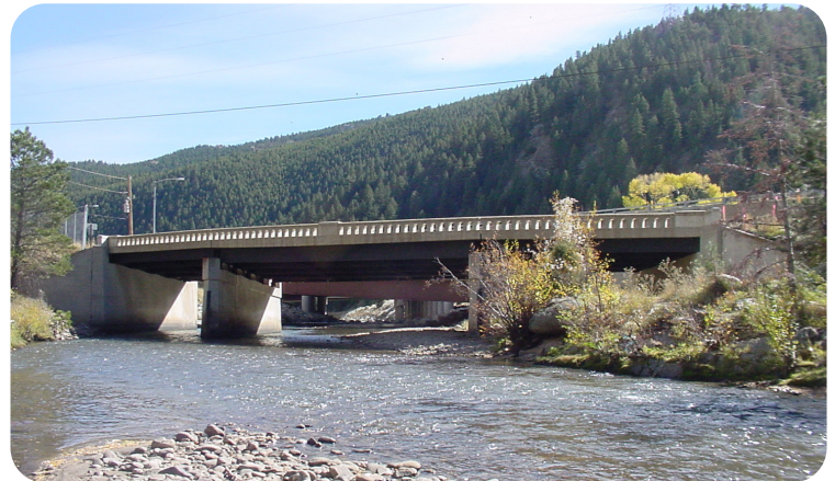
Image 13. I-70 Frontage Road over Clear Creek (F-15-D)
