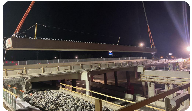
Image 17. Girder Installation for I-70 ML over W. 32nd Ave
