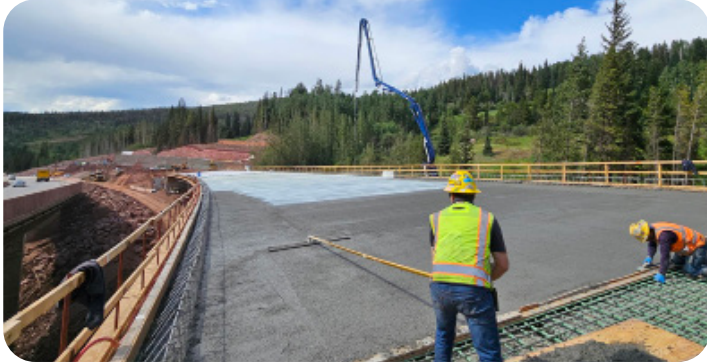
Image 14. New Bridge Deck of the future I-70 WB over Polk Creek
