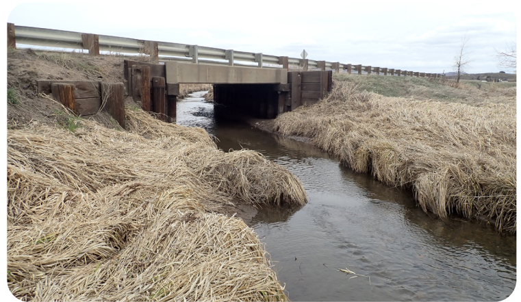
Image 9. US 40 ML over Shelton Ditch (C-08-A_Minor)
