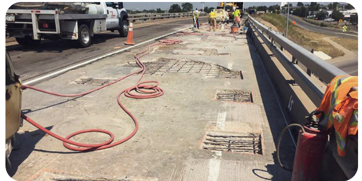
Image 15. Emergency Repairs on I-270
