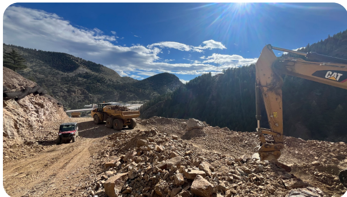
Image 11. Excavation for the Floyd Hill Project
