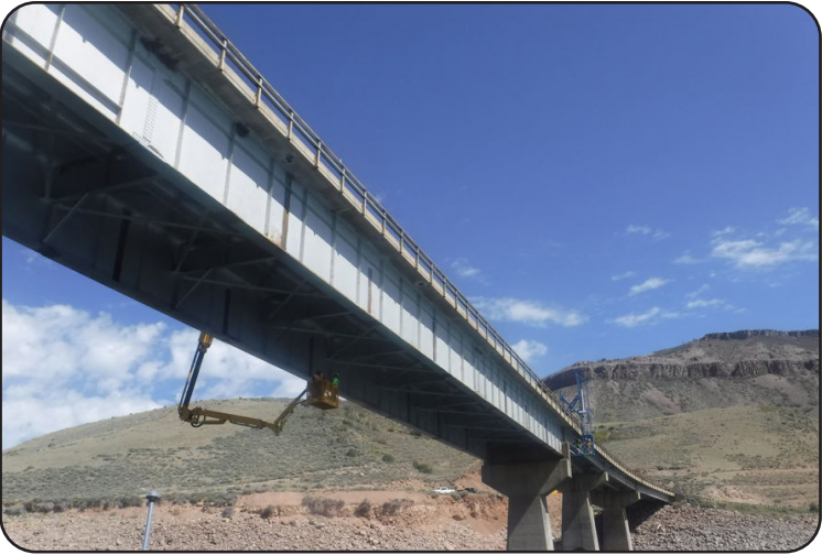
Image 7. Substructure of US 50 ML over Blue Mesa Reservoir
