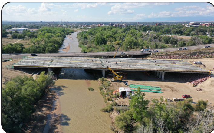
Image 10. Construction on the New Pueblo Freeway Project
