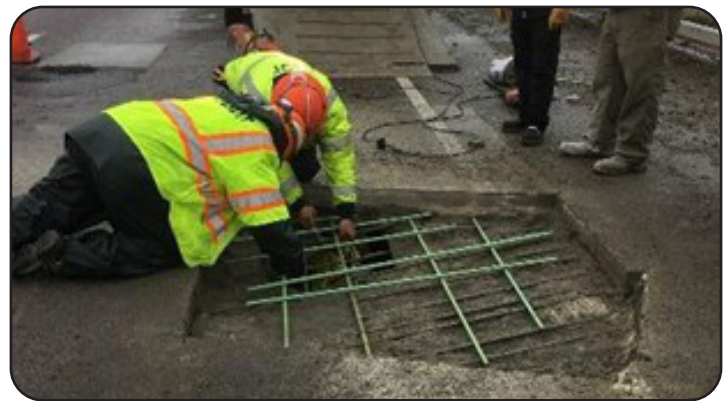
Image 14. Repairs on I-270
