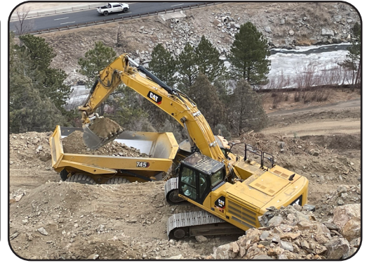
Image 7. CP #3 Saddle Cut Excavation
