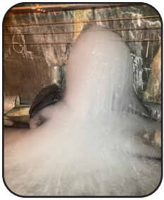
Image 16. Ice Build-up on the EJMT Liner
