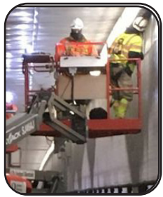
Image 17. Repairs on the EJMT Lighting
