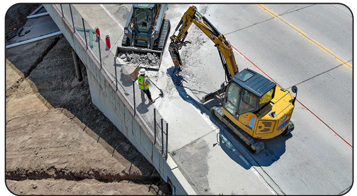
Image 14. Repairs on I-270
