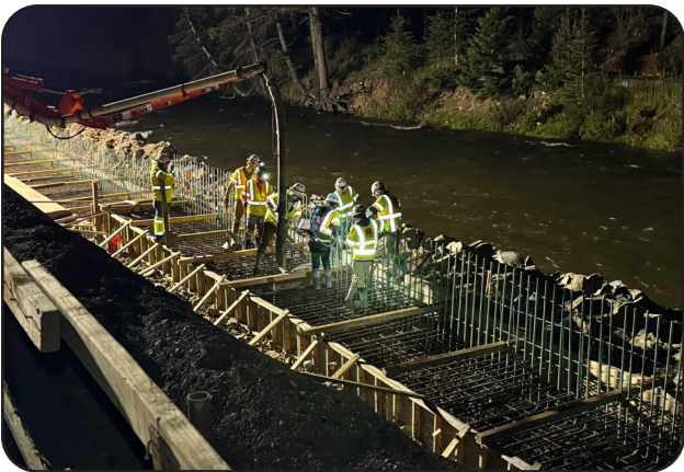
Image 1. Night Work on Floyd Hill
