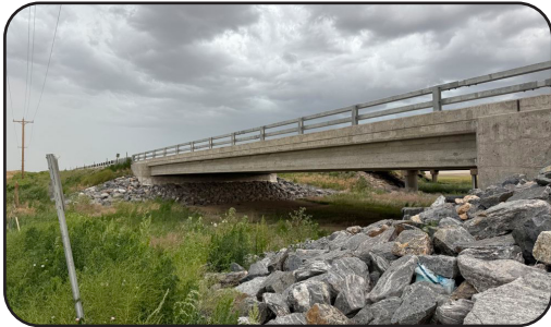
Image 3. I-70 Service Road over Draw
