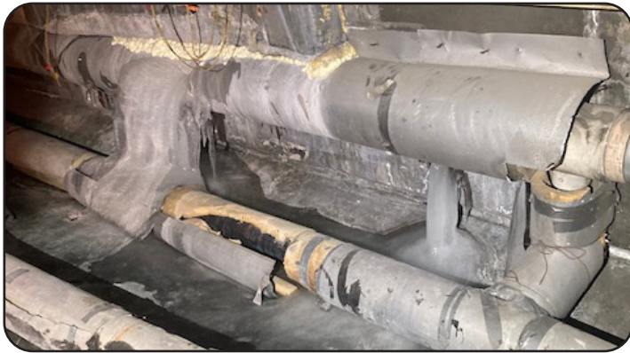
Image 16. Ice Buildup on the EJMT Plenum Liner
