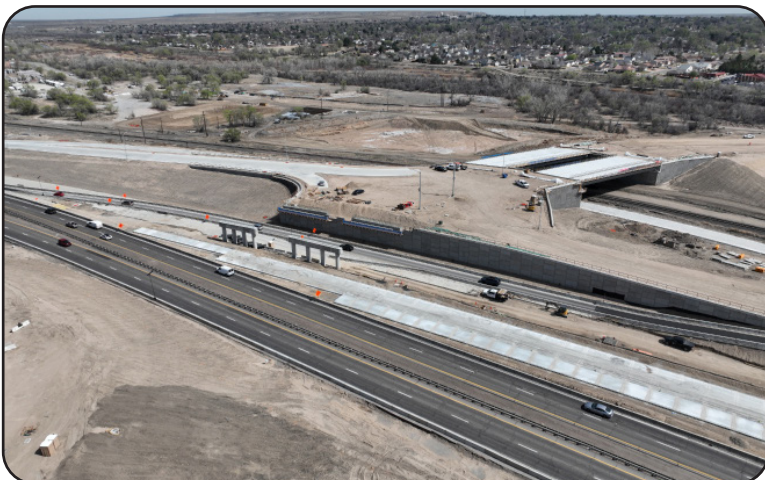
Image 14. Construction on the New Pueblo Freeway Project
