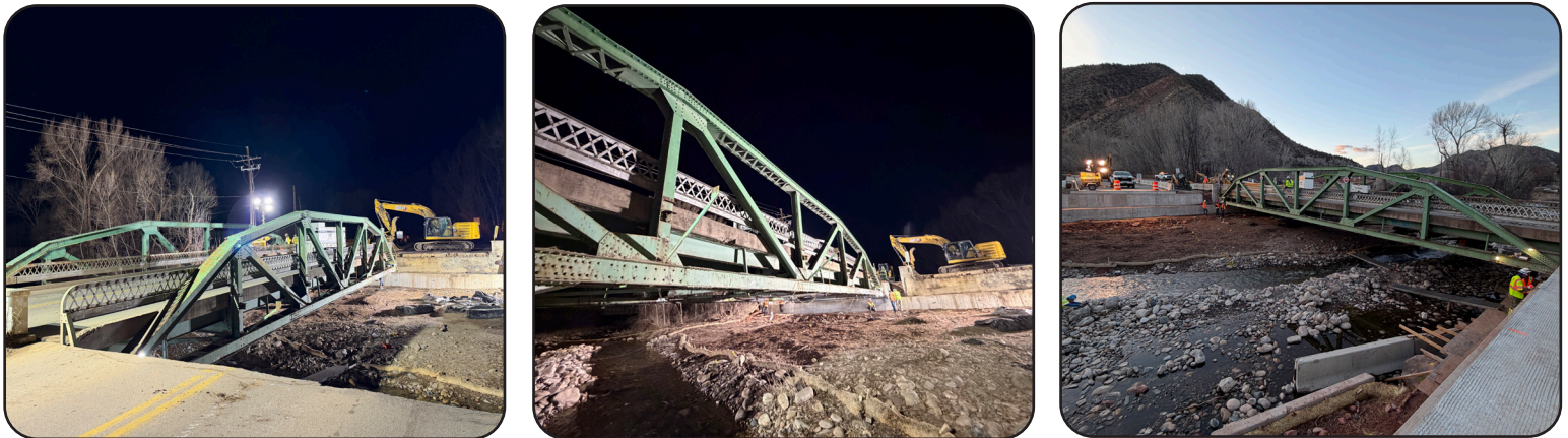
Image 1-3. Progression of the US 6 over Elk Creek Bridge Slide
