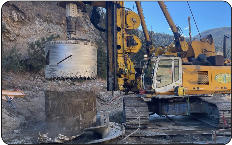
Image 15. Drilled Shaft for the Future I-70 over Clear Creek Structure
