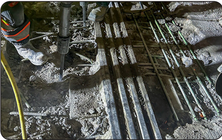
Image 18. Repairs on I-270
