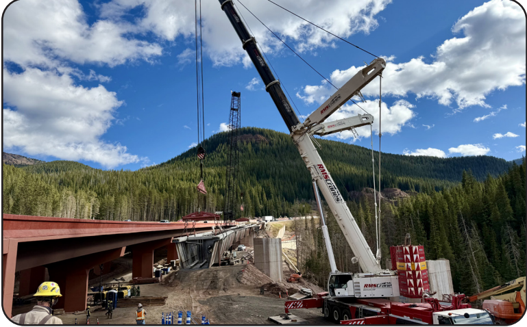
Image 17. Deck Work for the New I-70 EBND Structure
