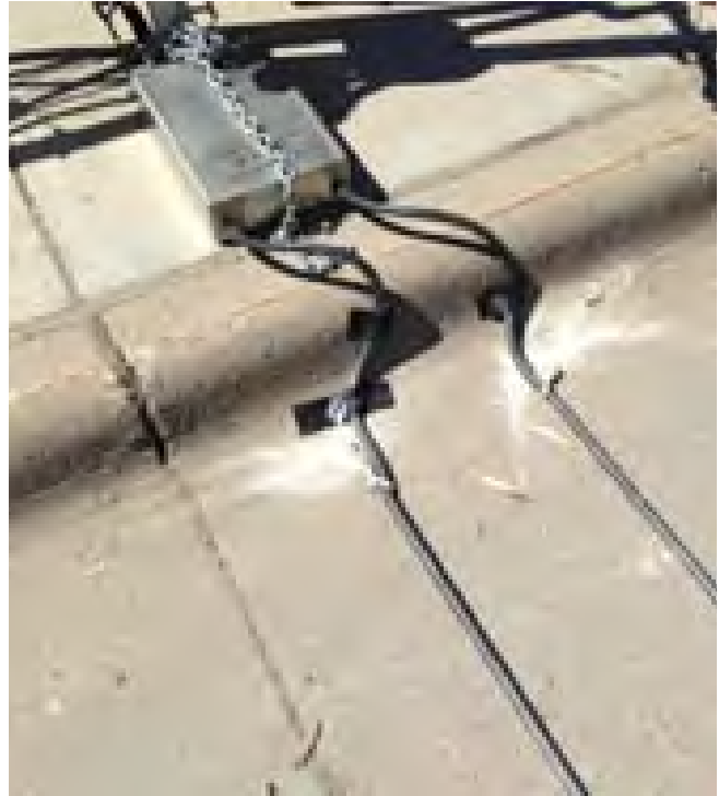
Figure A-4. Pneumatic Tube Installation
