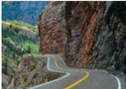
Highway with no Shoulder
