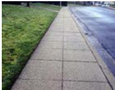
Narrow, Attached Sidewalk
