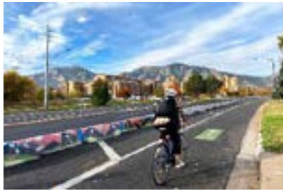
Bike Lane with a Protective Barrier from Traffic
