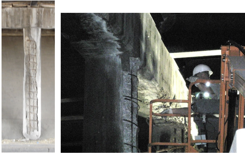
Fig. 16.12(D)-3 Photos showing column damage and repair process
