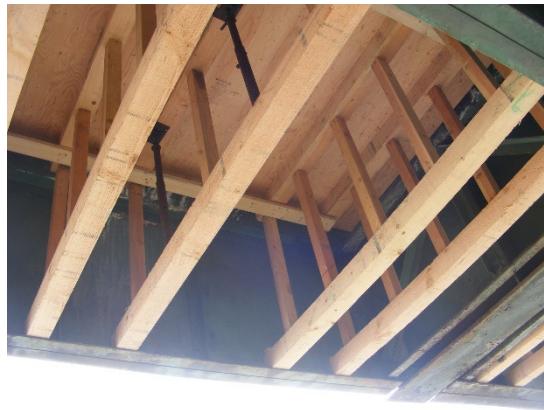
Fig. 16.12(I)-2 Photo of Deck Falsework
