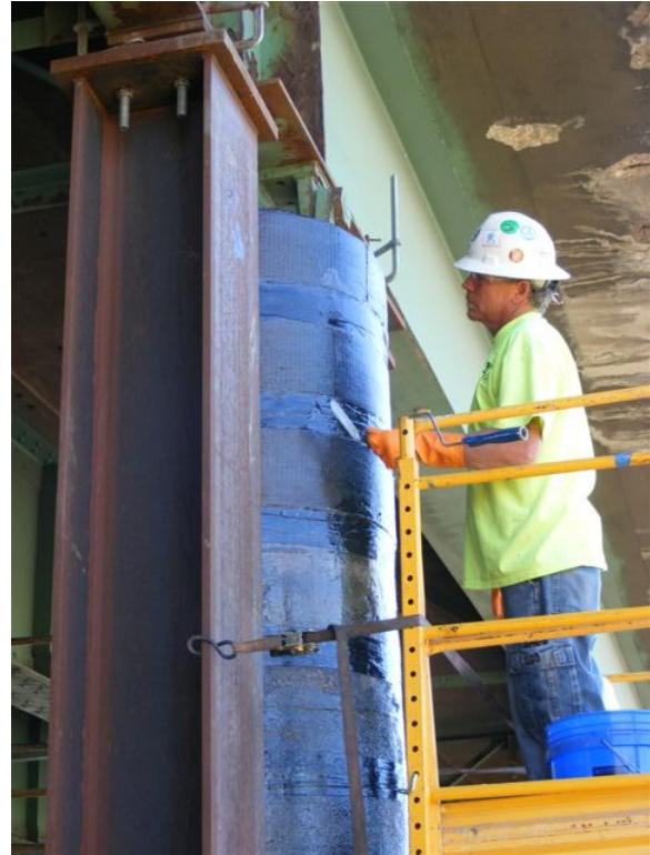
Fig. 16.12(D)-7 Photo of Fiber Wrap
