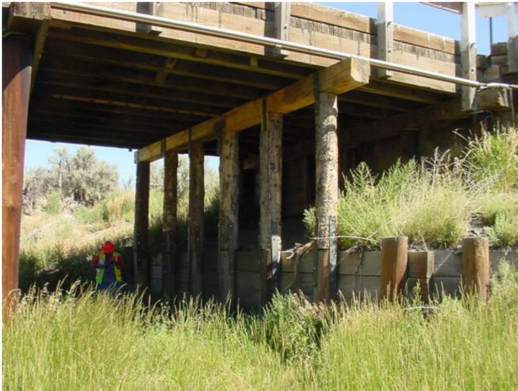
Fig. 16.12(H)-9 Photo of New Timber Bent
