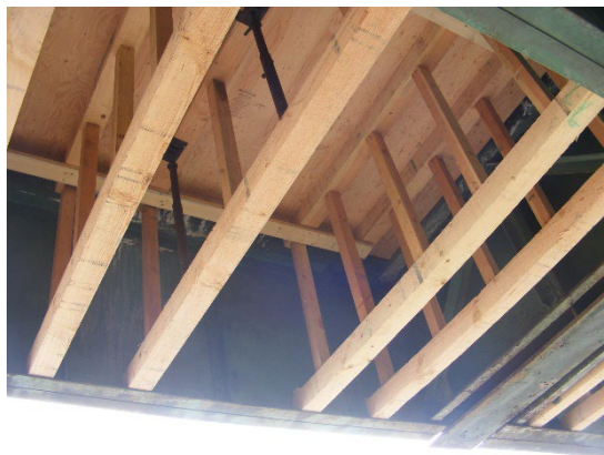
Fig. 16.12(I)-2 Photo of Deck Falsework
