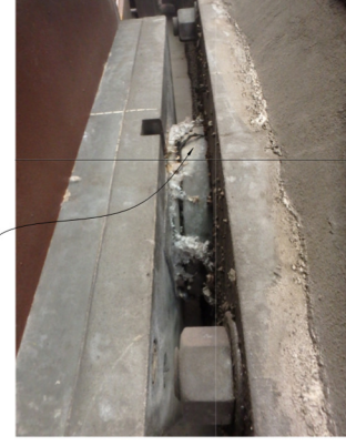
Pot Bearing to be replaced
