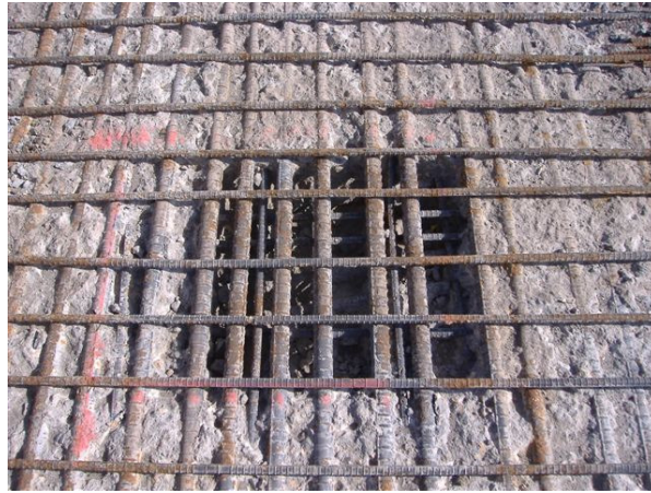
Fig. 16.12(C)-5 Close-up Photo of Deck Rehabilitation
