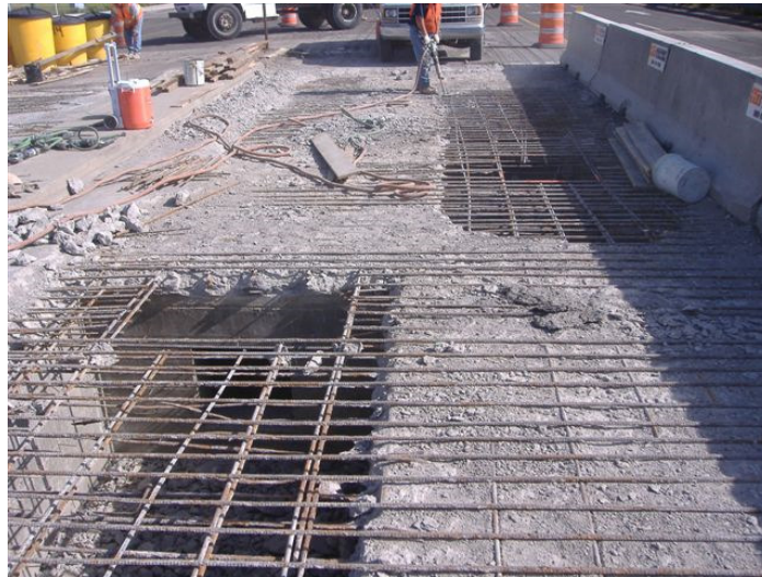
Fig. 16.12(C)-6 Photo of Deck Rehabilitation (Removals approaching critical levels)
