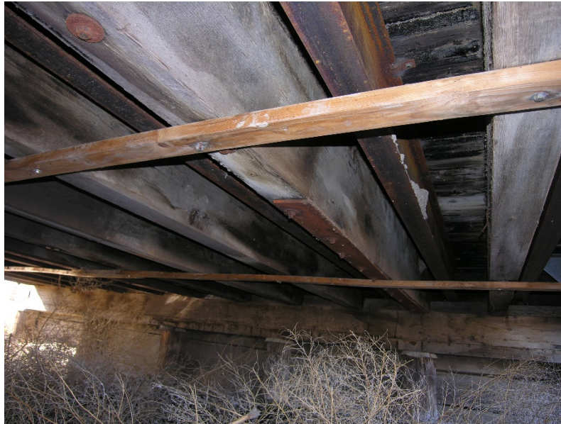
Fig. 16.12(H)-5 Photo of Added Steel Girder and Grader Blade on Timber Girder
