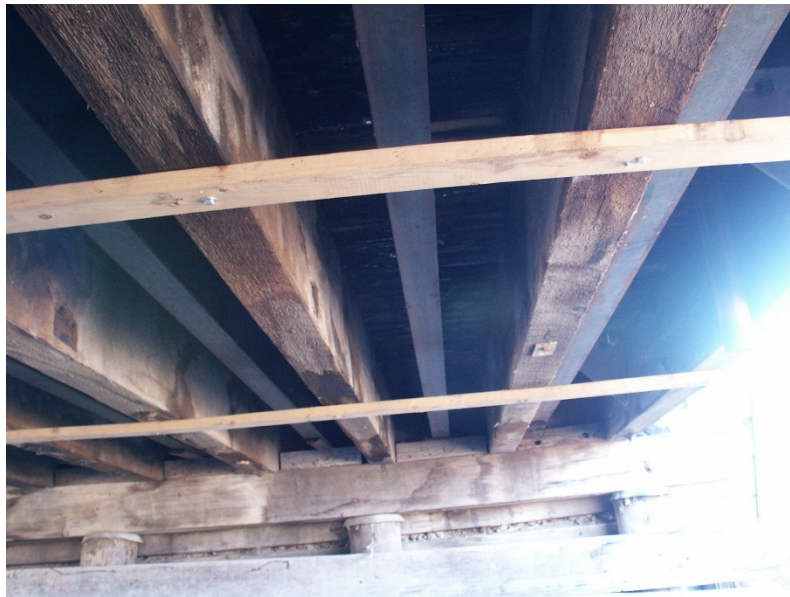
Fig. 16.12(H)-4 Photo of steel girders added to a Timber Bridge
