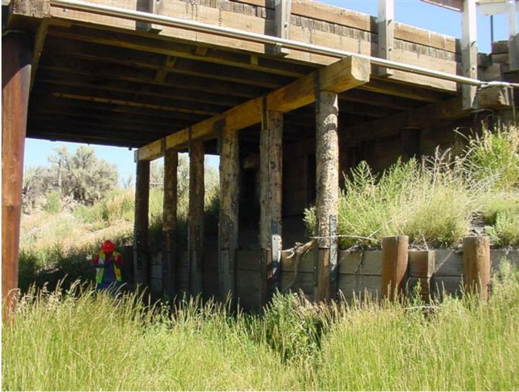
Fig. 16.12(H)-9 Photo of New Timber Bent
