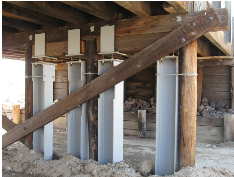
Fig. 16.12(G)-6 Photo of Adding Columns to a Pile
