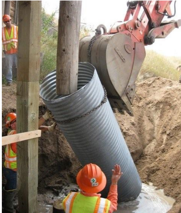
Fig. 16.12(G)-2 Photo of Timber Pile/Column Repair in progress
