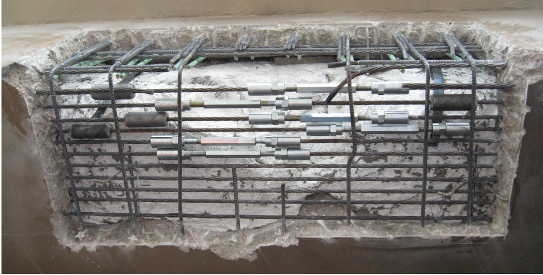
Fig. 16.12(E)-5 Photo of Precast Girder repair in progress
