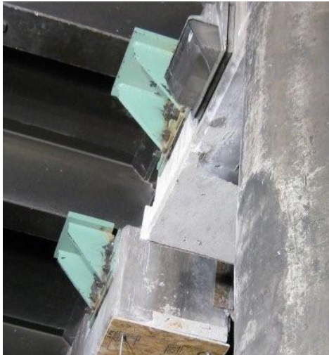
Fig. 16.12(F)-5 Front Side of Corbel
