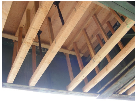
Fig. 16.12(I)-2 Photo of Deck Falsework
