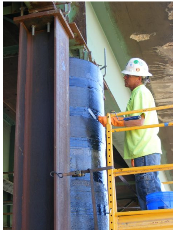
Fig. 16.12(D)-7 Photo of Fiber Wrap
