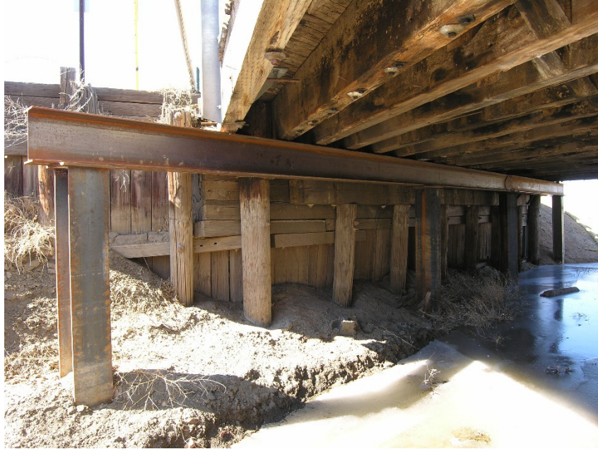
Fig. 16.12(H)-7 Photo of New Support Bent near Abutment
