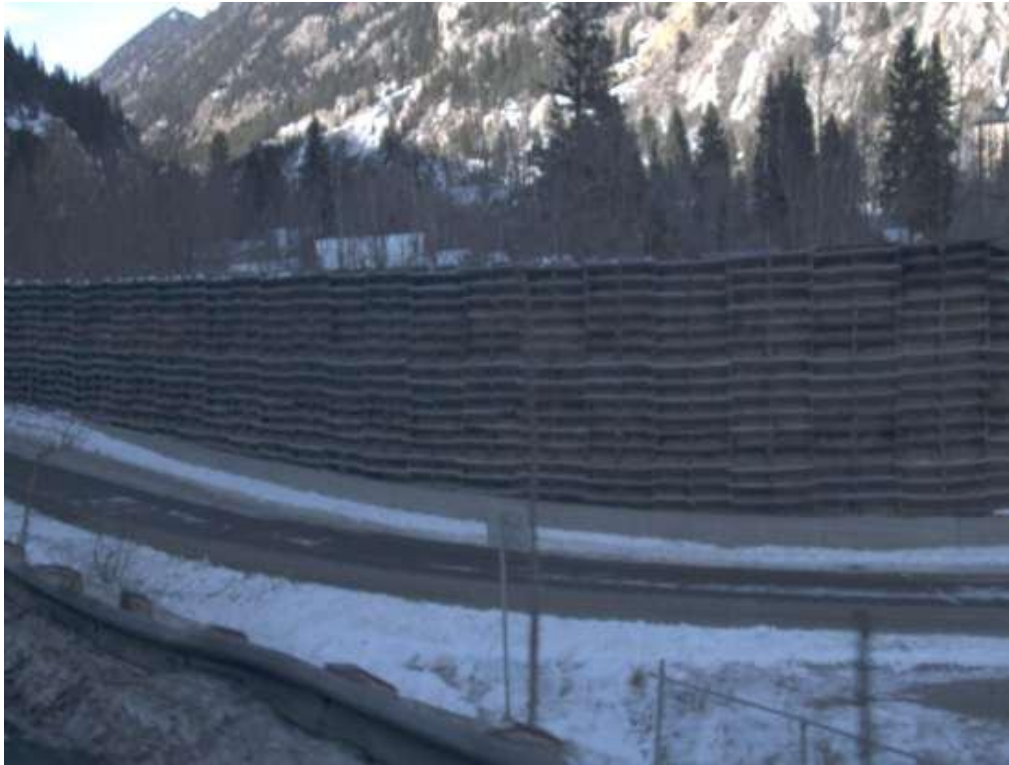
Fig. 15.1.13-7 Miscellaneous Sound Barrier Example
