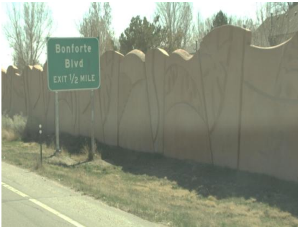
Fig. 15.1.13-8 Miscellaneous Sound Barrier Example 2
