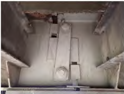
Overview of Girder 2B pin and hanger assembly and splice at Pier 2
