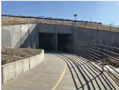
Culvert outlet looking east
