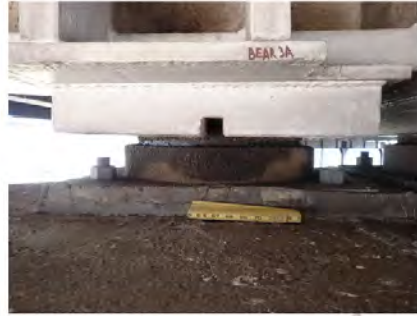
Overview of Bearing 3A 6/27/2025 12:00:00 AM
