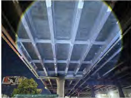
Superstructure looking east - Span 8
