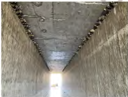
Culvert general looking east
