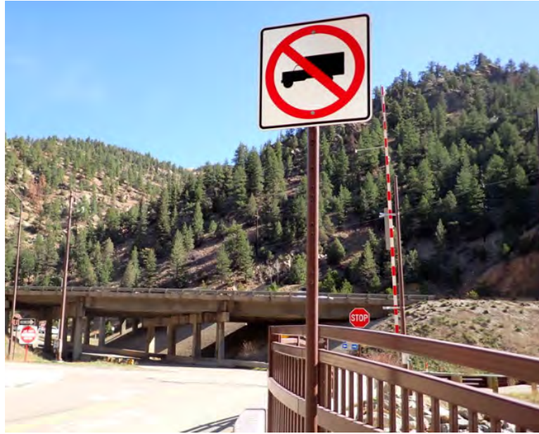
Figure 7. "No Trucks" (MUTCD R5-2) sign erected at Off-System structure (Example 3)
