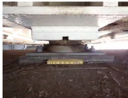
Overview of Bearing 2C 6/27/2025 12:00:00 AM
