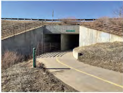
Culvert inlet looking west
