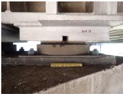
Overview of Bearing 3B 6/27/2025 12:00:00 AM
