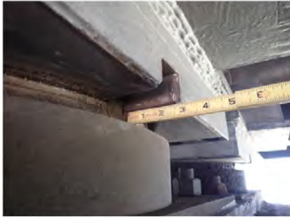
3 inches to edge of bearing plate on east side of Bearing 3B 6/27/2025 12:00:00 AM
