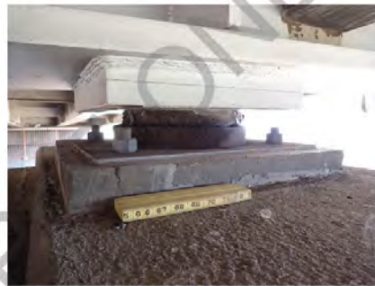
Overview of Bearing 2A 6/27/2025 12:00:00 AM
