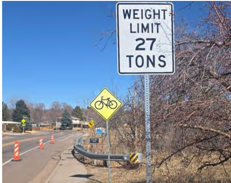
Figure 5. Load posting sign erected at Off-System structure (Example 1)
