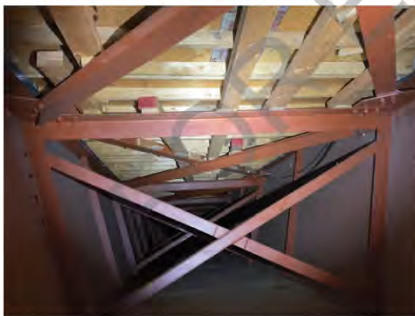
Timber forms in Girder A at the deck bottom.
