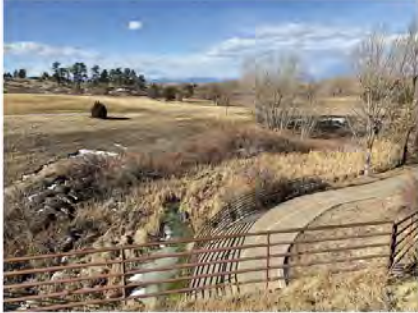
Channel looking west downstream
