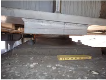
Overview of Bearing 2D 6/27/2025 12:00:00 AM
