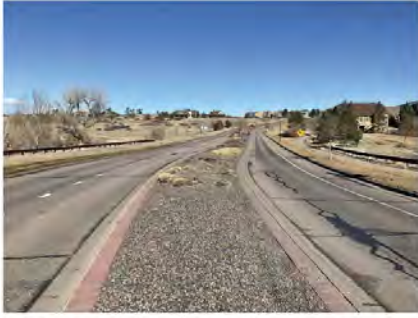
Roadway looking north
