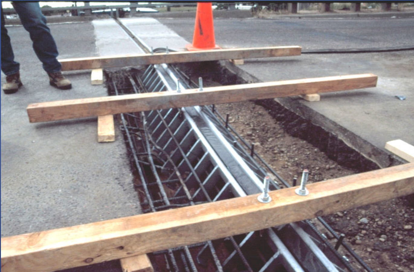
INADEQUATE REBAR
