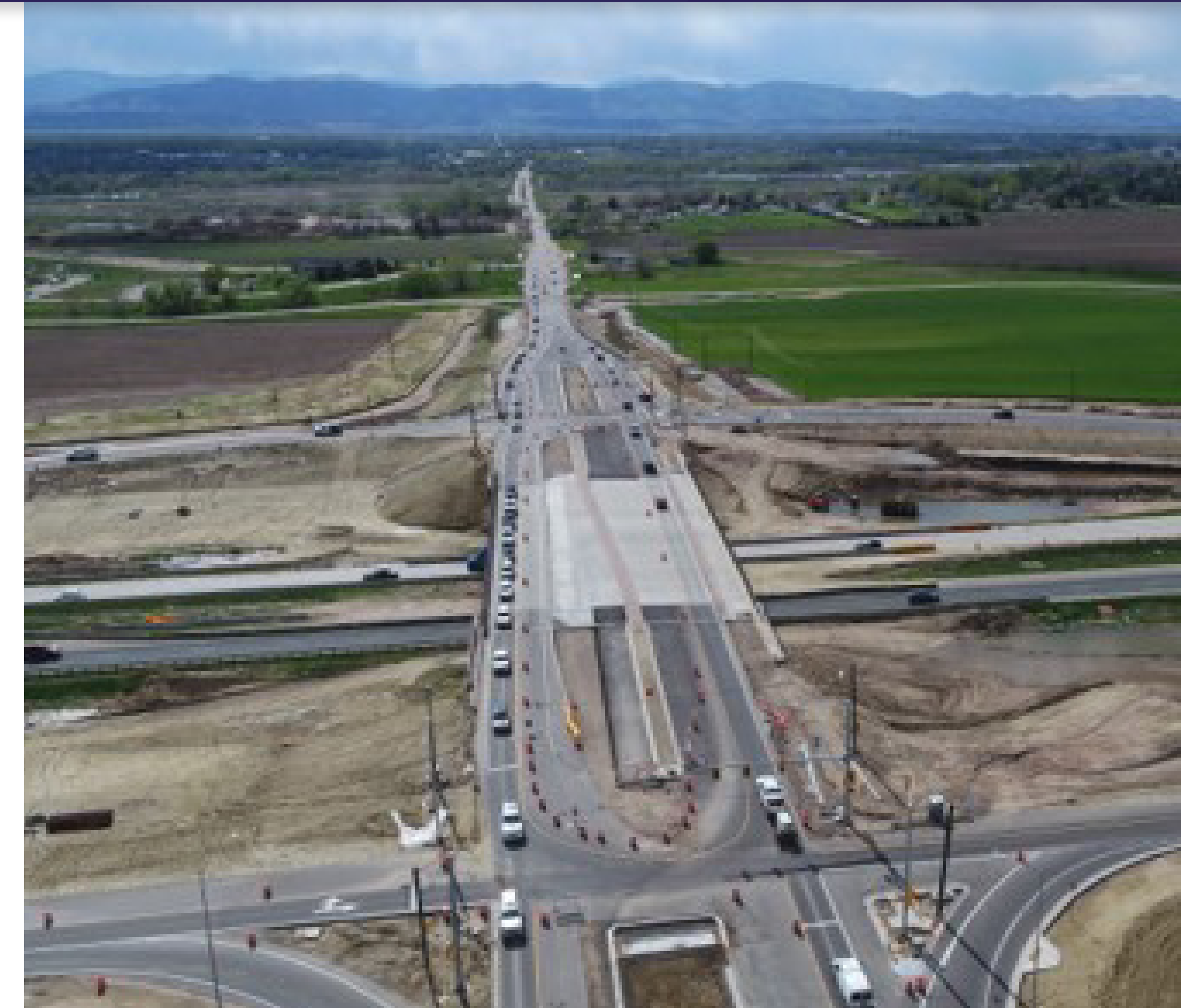
Prospect Road - After
