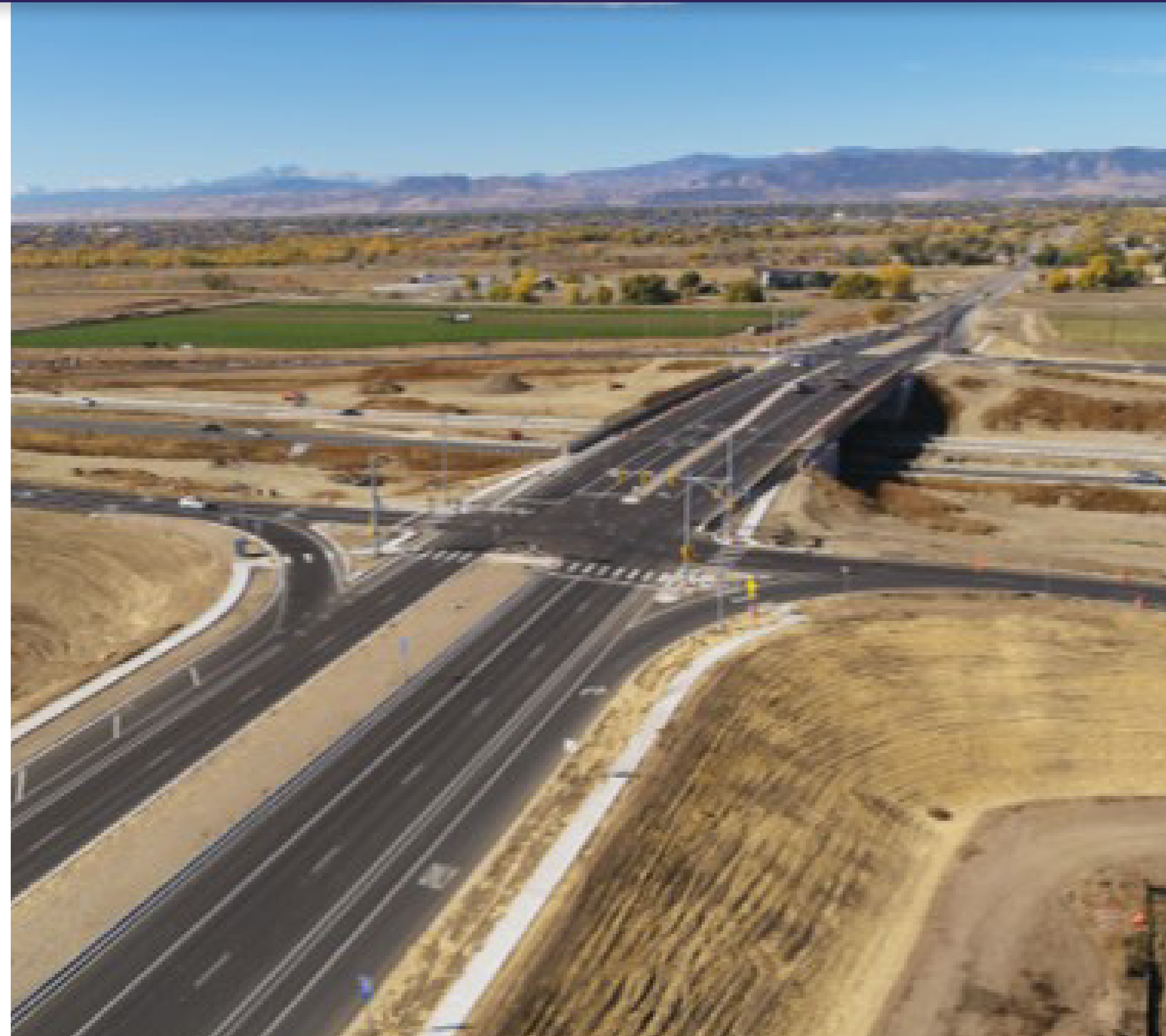
Prospect Road - After
