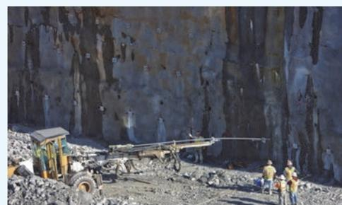
*Rock wall stabilization for future retaining wall system*
