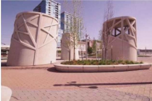
*Ventilation towers for underground bus terminal located in LRT station plaza*
