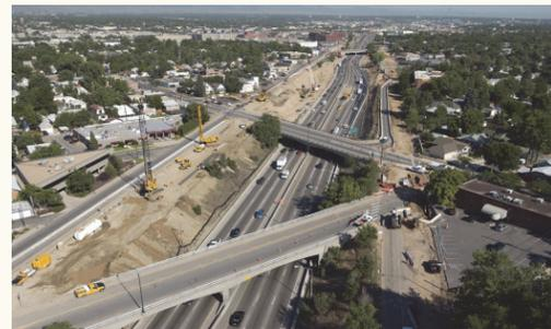
*Beginning of drilled shaft installation for walls in the Narrows*
