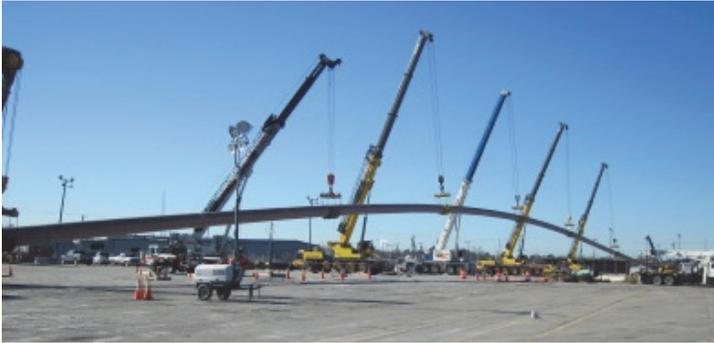
*The 4,500 linear ft. subaqueous section of the new 36-in. water main was assembled on the Portsmouth side of the river and installed in one weekend, minimizing impact to the public*
