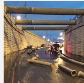
*Jorgensen installing pumps to remove flooding water during the 2015 event*
