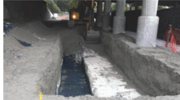
*Ground improvements beneath First Avenue adjacent to existing columns were designed to account for local seismic activity*
