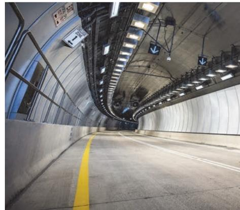
*Interior of tunnel with jet fans used maintain air quality & control airflow*
