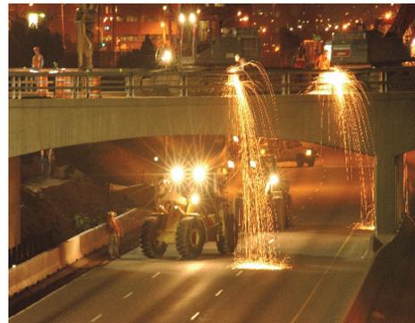
*“Washington Street Bridge – removing metal railing prior to structure demolition*
