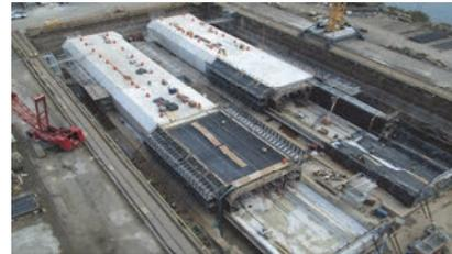
*Precast tunnel segment are built quickly at the Sparrows Point dry dock*
