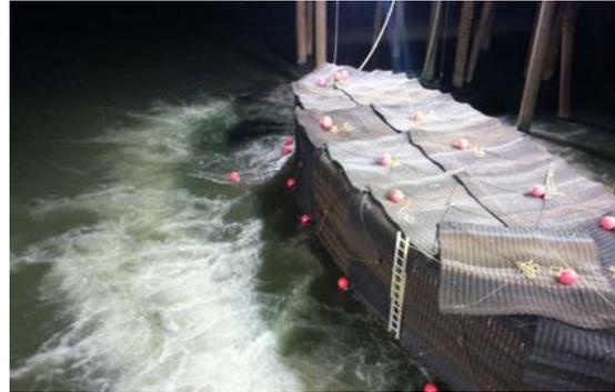
*Kiewit implemented bubble curtains, fish deterrents, and comprehensive monitoring to protect aquatic wildlife during the demolition of large piers on the existing Port Mann bridge*
