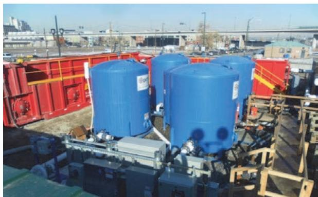
*Treatment system for handling the contaminated dewatering*
