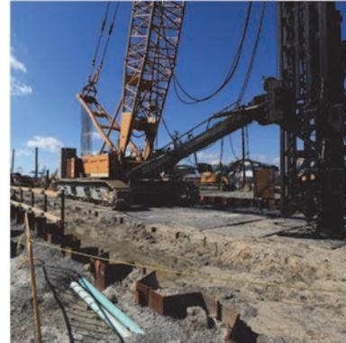
*Noise and vibrations were monitored during concrete pile driving operations to limit noise impact to the surrounding community*
