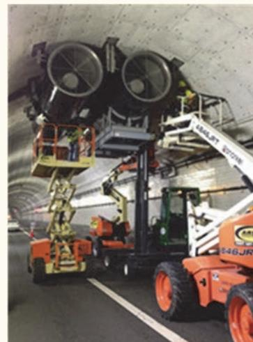
*New jet fans installed in the existing tunnels are an upgrade to meet current NFPA fire life safety requirements*
