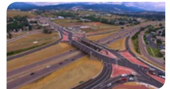
Constructing the I-25/Fillmore Diverging Diamond Interchange while maintaining traffic flow presented project phasing challenges. To deliver the project on time, SEMA proposed adjustments to the original 16-phased sequence plan, including implementing two fast-track weekend closures when traffic was lighter, that cut approximately two months from the schedule.
