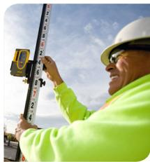
Process control teams perform survey control check (top) and stone matrix asphalt density test (bottom).
