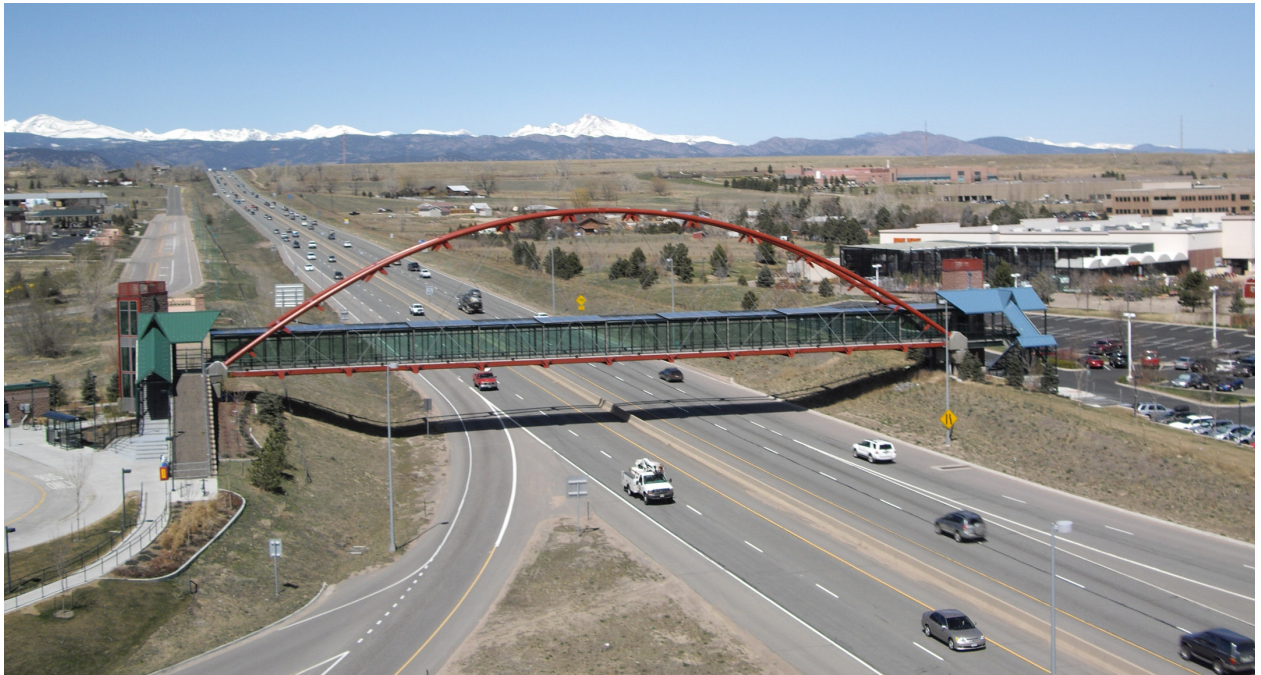
Louisville/Superior pedestrian bridge provides connectivity to BRT stations
