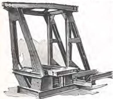
hoist, drum or traction, is taken by the entire single-unit frame.
