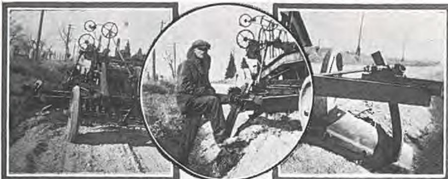
*Showing new shoulder blade attachment on Russell Patrol Motor grader working on Weld county paved roads.*
