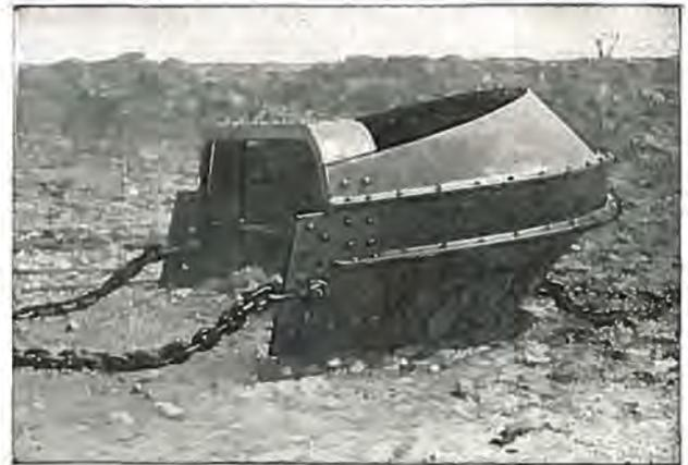
The mold board action of the cutting edge makes the Crescent Scraper a powerful digger. Will excavate hard packed gravel and large boulders. Requires less power than other types.
