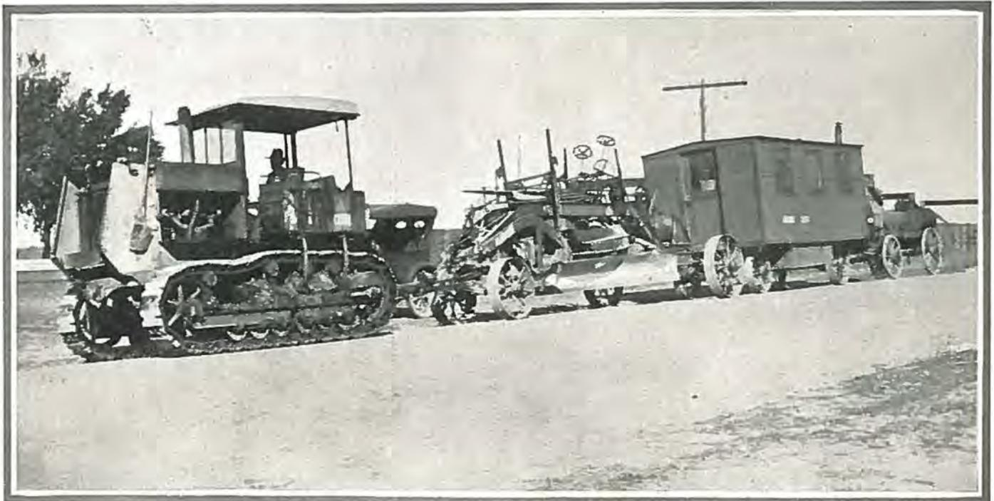
A "train" of road machinery on the way... In this modern train the tractor serves as the locomotive, pulling a grader, cook house and supply wagon.
