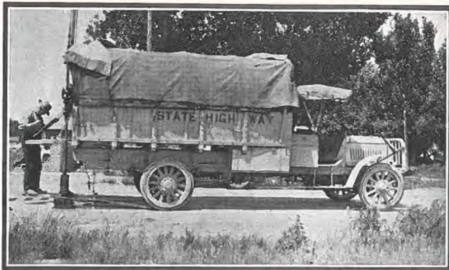
The State highway department new core drill machine, which is used to detect faulty concrete pavement—Foreman Skerret is shown operating machine.
