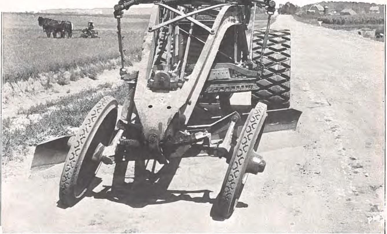
The chief feature of the 15-30 Austin International Motor Grader is that it has weight and power enough to cut right down to the bottom of the corrugations of a badly rutted gravel road, for which reason it can rightly be called a reconstruction as well as a maintenance machine.
