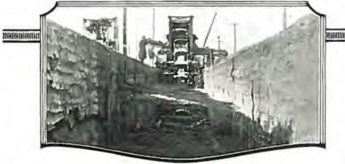
The Rotary Auxiliary Cutter enables every Buckeye to dig many widths of trench. Therefore, any Buckeye can do the work of several ordinary excavators.
