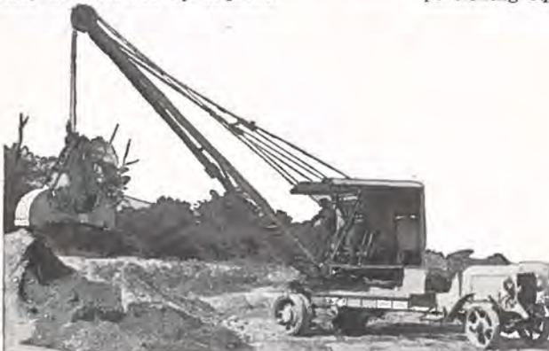
*New Model P & H Truck Crane manufactured by the Harnischfeger Corporation.*
