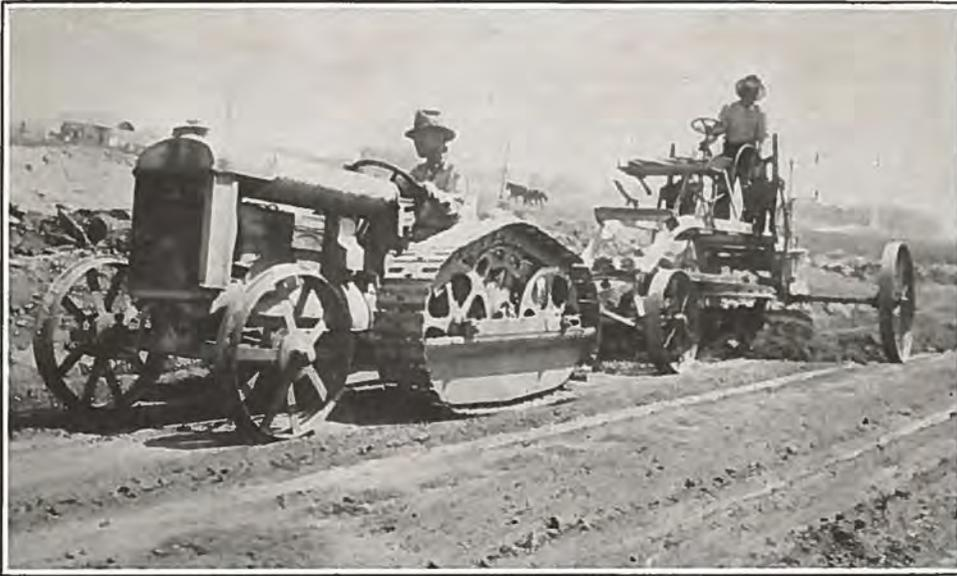
Knorr Construction Company using 7 foot 3 blade behind the Fordson in road construction work near Denver. This company used two of these units this summer in order to cut their operating costs.
