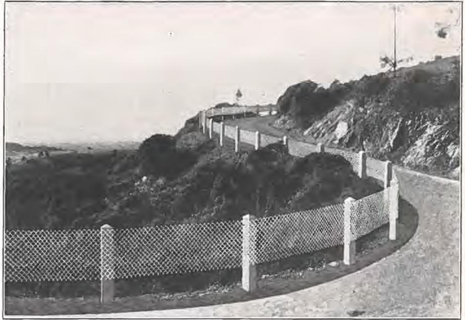
*Cyclone Road Guard—the new type roadway fence designed and built sufficiently strong to catch cars that swerve from the road. There is no record of this fence ever having been broken through.*
