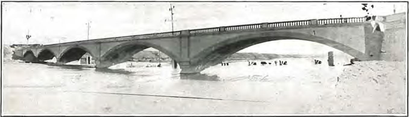
One of the longest concrete bridges in Colorado is the Huerfano River highway structure shown in the accompanying photograph. This huge bridge has five spans, each 80 feet in length, making the entire length of the structure 400 feet.
