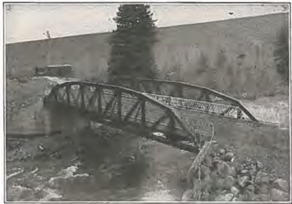
100 ft. Riveted Low Truss Span, Dillon, Colo.
