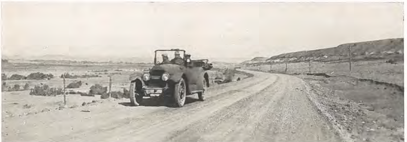
Gravel surfaced state highway located north of Salida in Chaffee County.
