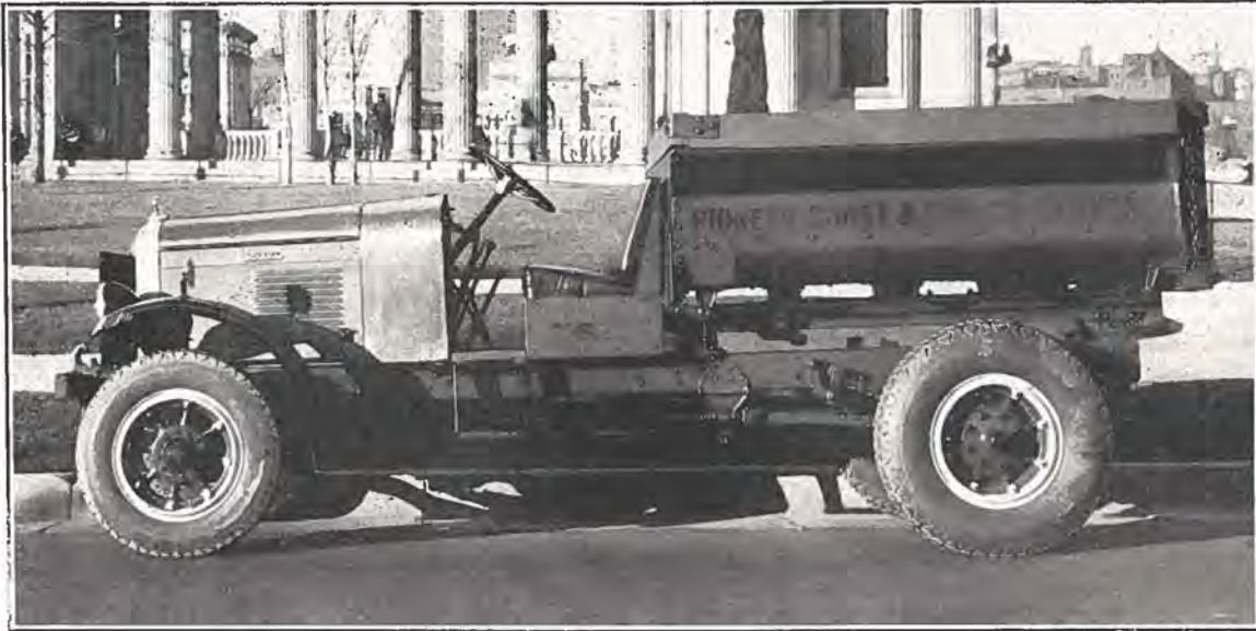
Indiana Model 615-A, with hydraulic hoist and dump body—one of a fleet owned by Pioneer Construction & Engineering Co., Denver.
