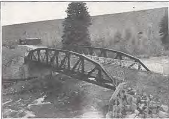
100 ft. Riveted Low Truss Span, Dillon, Colo.
