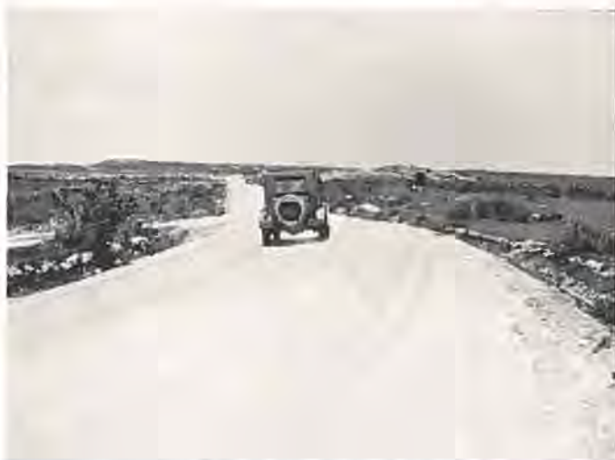
An example of limestone road construction is given in this photograph taken by M. W. Bennett. The scene is west of Pueblo, toward Florence. This highway has attracted attention of road builders, as it is almost as hard as concrete.
