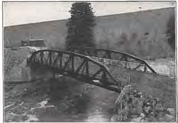
100 ft. Riveted Low Truss Span, Dillon, Colo.
