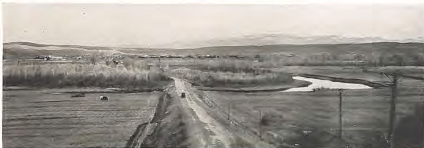
A view of a new road constructed by the state south of Craig, showing a stretch of the Yampa River. Photo by H. L. Jenness, Division Engineer.
