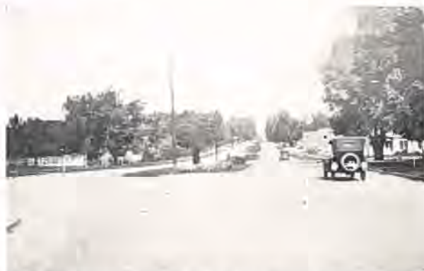
View of paved street in Fort Collins connecting with state highway
