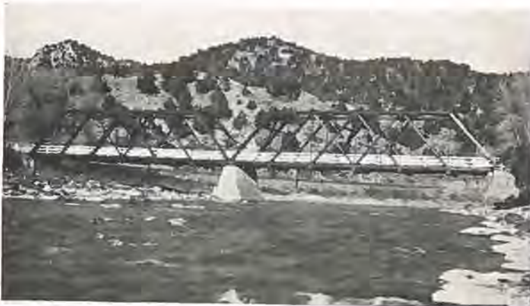
Bridge over the Eagle River at Wolcott, connecting State Road No. 11 with U. S. Highway No. 40.
