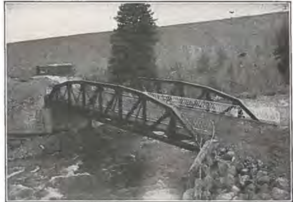
100 ft. Riveted Low Truss Span, Dillon, Colo.
