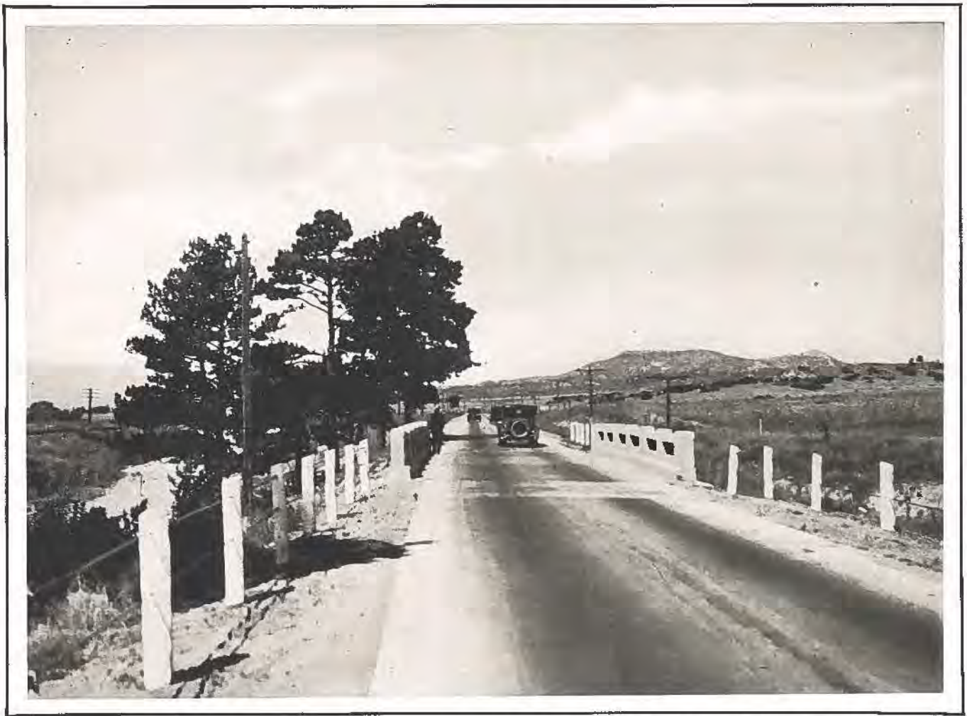
A section of the concrete paved Denver-Colorado Springs Road, in Douglas County
