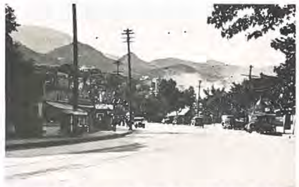
A section of the pavement on U. S. Highway No. 40 in town of Manitou.
