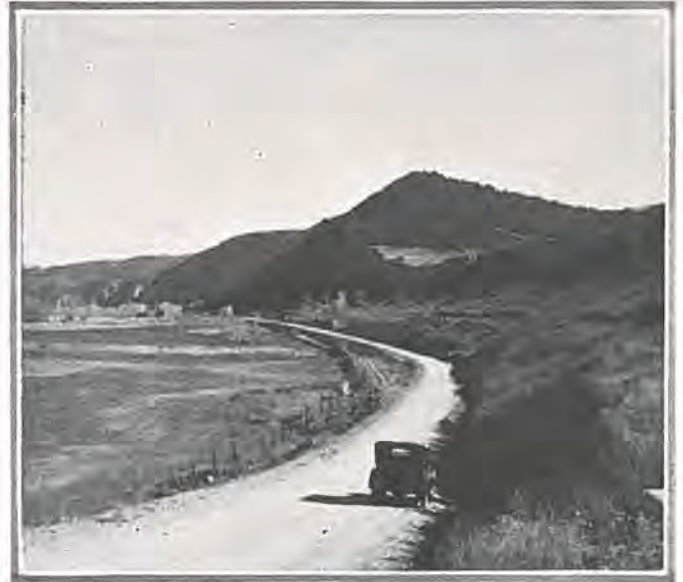
Scene on State Road No. 82, north of Carbondale, improved with state funds.
