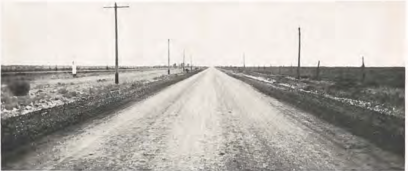
Another spot where the State Highway Department put an end to "Dusty Roads"—A view of the new oil surfaced highway near La Jara.
