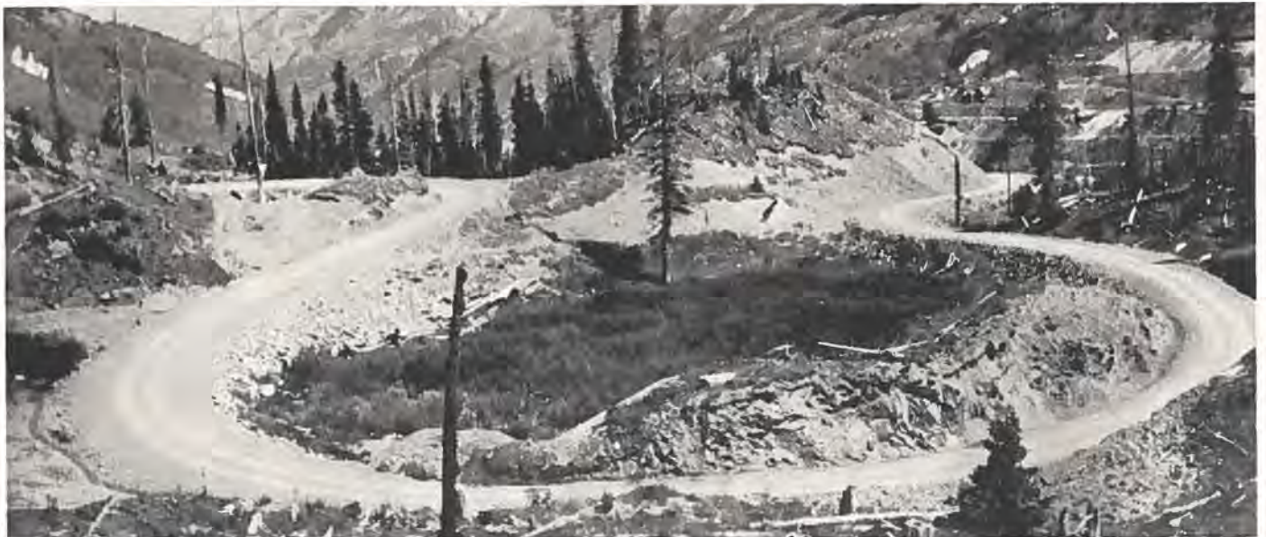
That popular song of another day, "Waltz Me Around Again, Willie," would be apt at this bit of state road on the Million Dollar Highway, extending from Ouray to Silverton, one of the world's scenic motor routes. This photograph taken by M. W. Bennett displays notable art with a camera and gives an idea of the width and ease with which the highway follows the old toll road built by that genius, Otto Mears. The scene is near Ironton, today a ghost city, but in early mining days a bustling camp. In the foreground are some of the workings from the Red Mountain group of mines.
