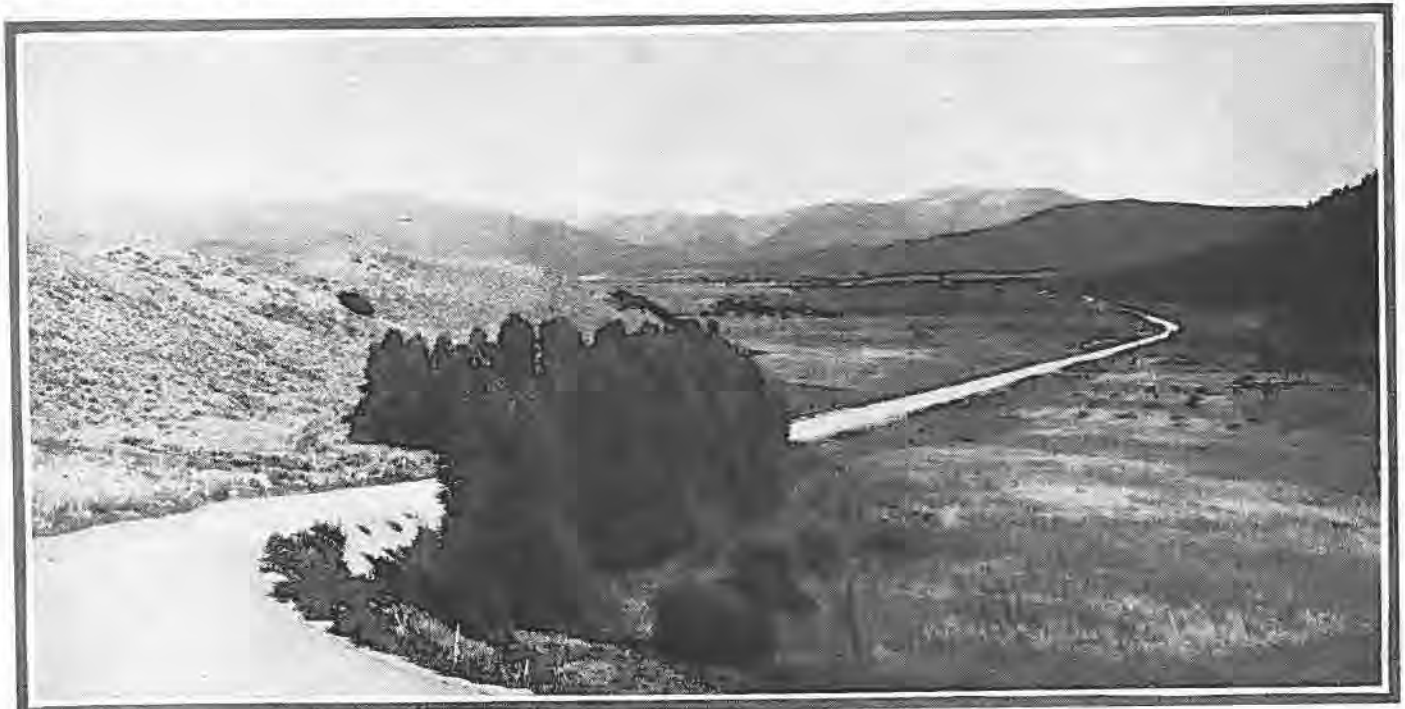
A beautiful gravel-surfaced highway, between Brookston and Milner in Routt County, constructed with Federal Aid funds.
