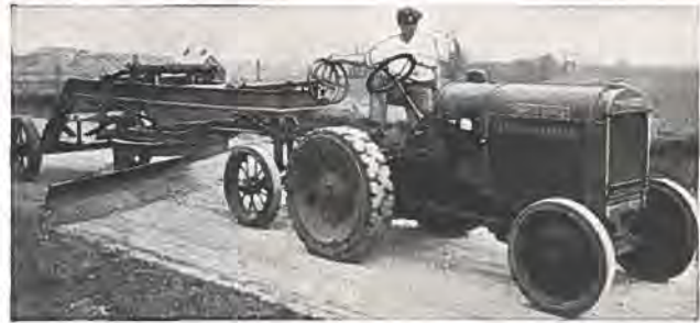
Above: The McCormick-Deering on highway maintenance
