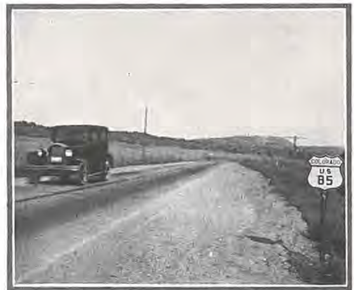
Stretch of concrete pavement south of Colorado Springs, recently completed with Federal Aid.
