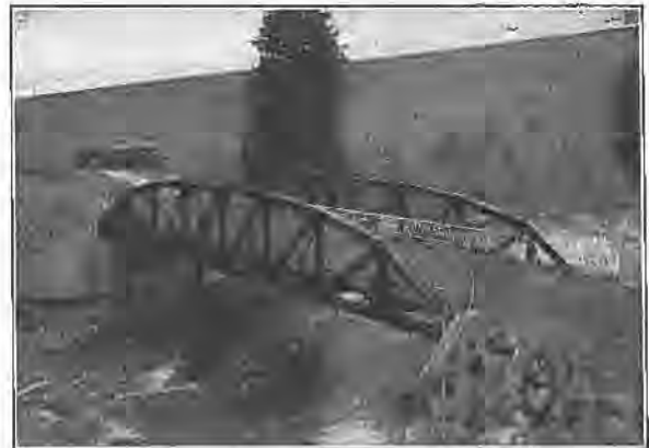
100 ft. Riveted Low Truss Span, Dillon, Colo.
