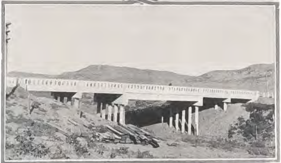
Stretch of new pavement and concrete bridge near Aguilar on State Road No. 1.
