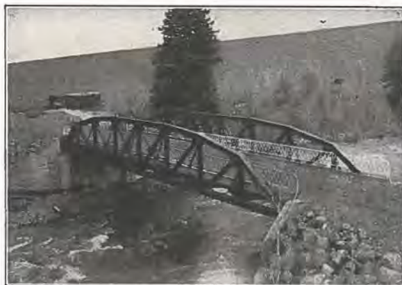
100 ft. Riveted Low Truss Span, Dillon, Colo.
