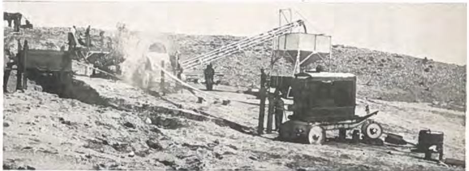
Cedar Rapids portable crusher outfit being used by Hamilton & Gleason on a state highway project near Lamar.
