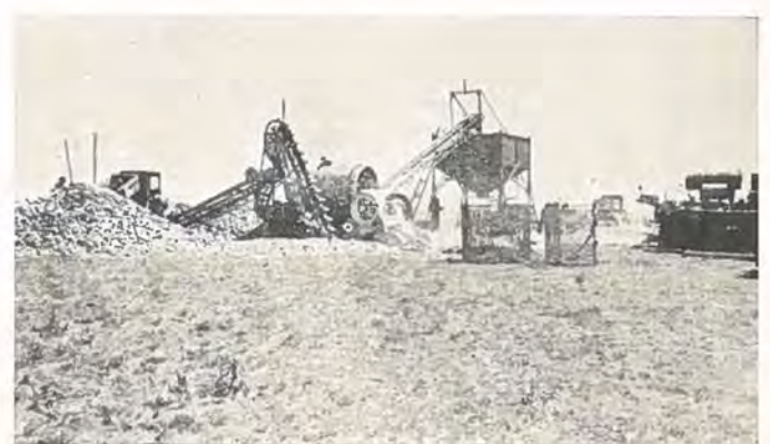
At left, showing tractor grader outfit turning oiled gravel; and at the right, rock crushing outfit preparing material for roadbed.
