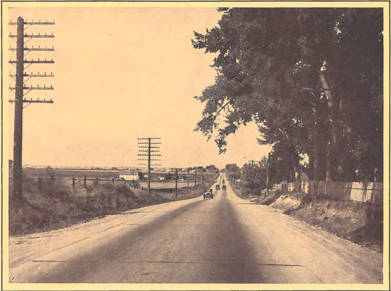
There is concrete all the way from Denver to Ft. Collins. This view was taken near Denver.
