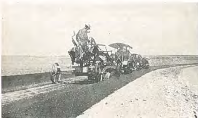
At left, showing tractor grader outfit turning oiled gravel; and at the right, rock crushing outfit preparing material for roadbed.
