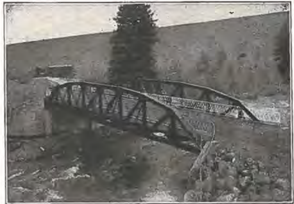
100 ft. Riveted Low Truss Span, Dillon, Colo.
