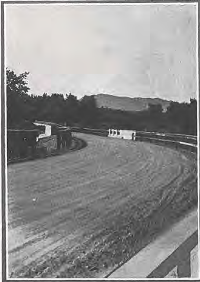
Section of Federal Aid highway located near Durango in La Plata county.
