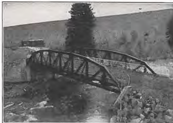
100 ft. Riveted Low Truss Span, Dillon, Colo.
