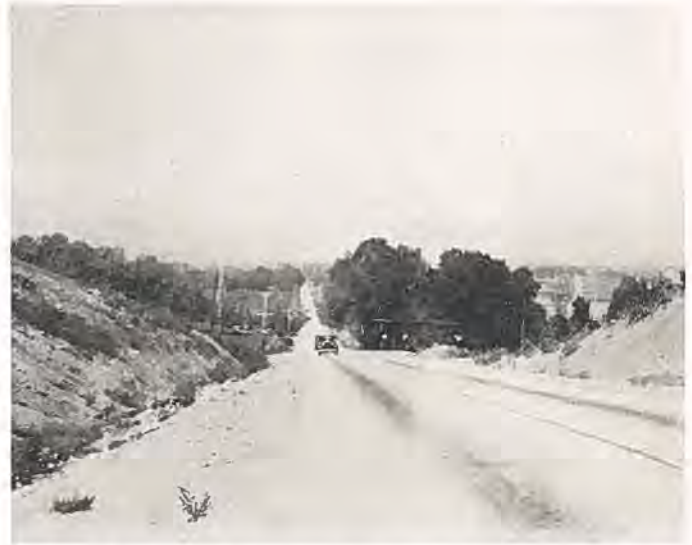
Showing stretch of new pavement entering Boulder, a Federal Aid project.
