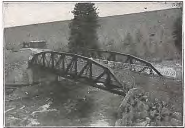
100 ft. Riveted Low Truss Span, Dillon, Colo.
