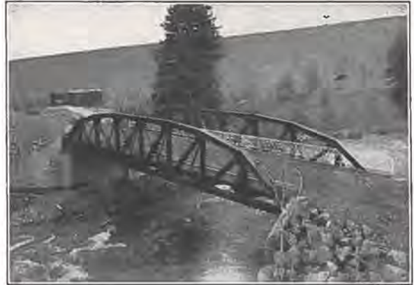
100 ft. Riveted Low Truss Span, Dillon, Colo.
