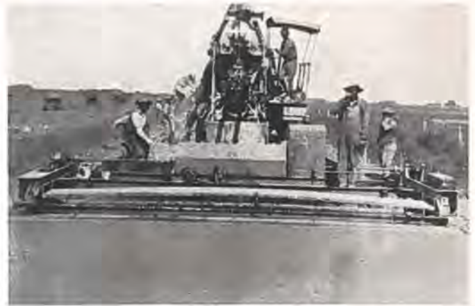
Ord Finishing Machine at work on Selander contract near Wiggins
