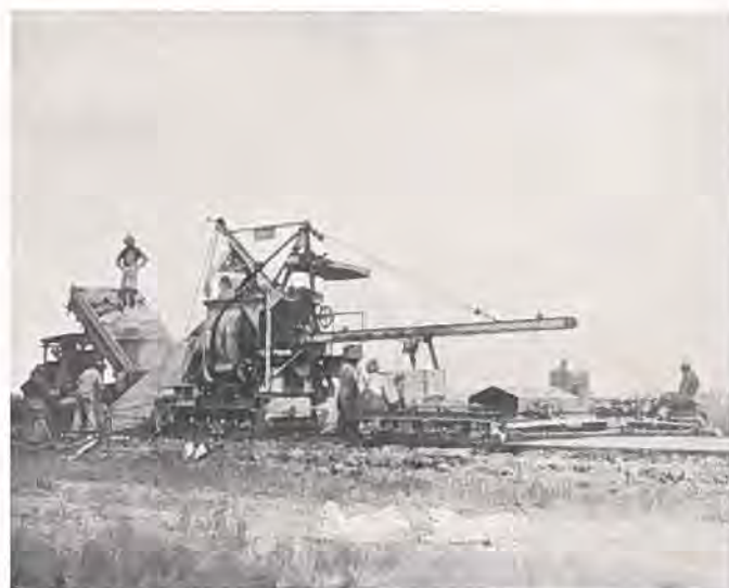
Typical concrete mixer outfit employed in construction of Colorado state roads.
