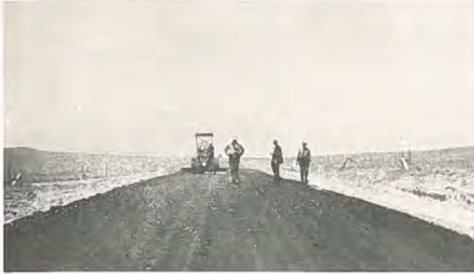
At left, final smoothing operation on oiled highway near Nunn; and at right, the road as it appears under traffic.
