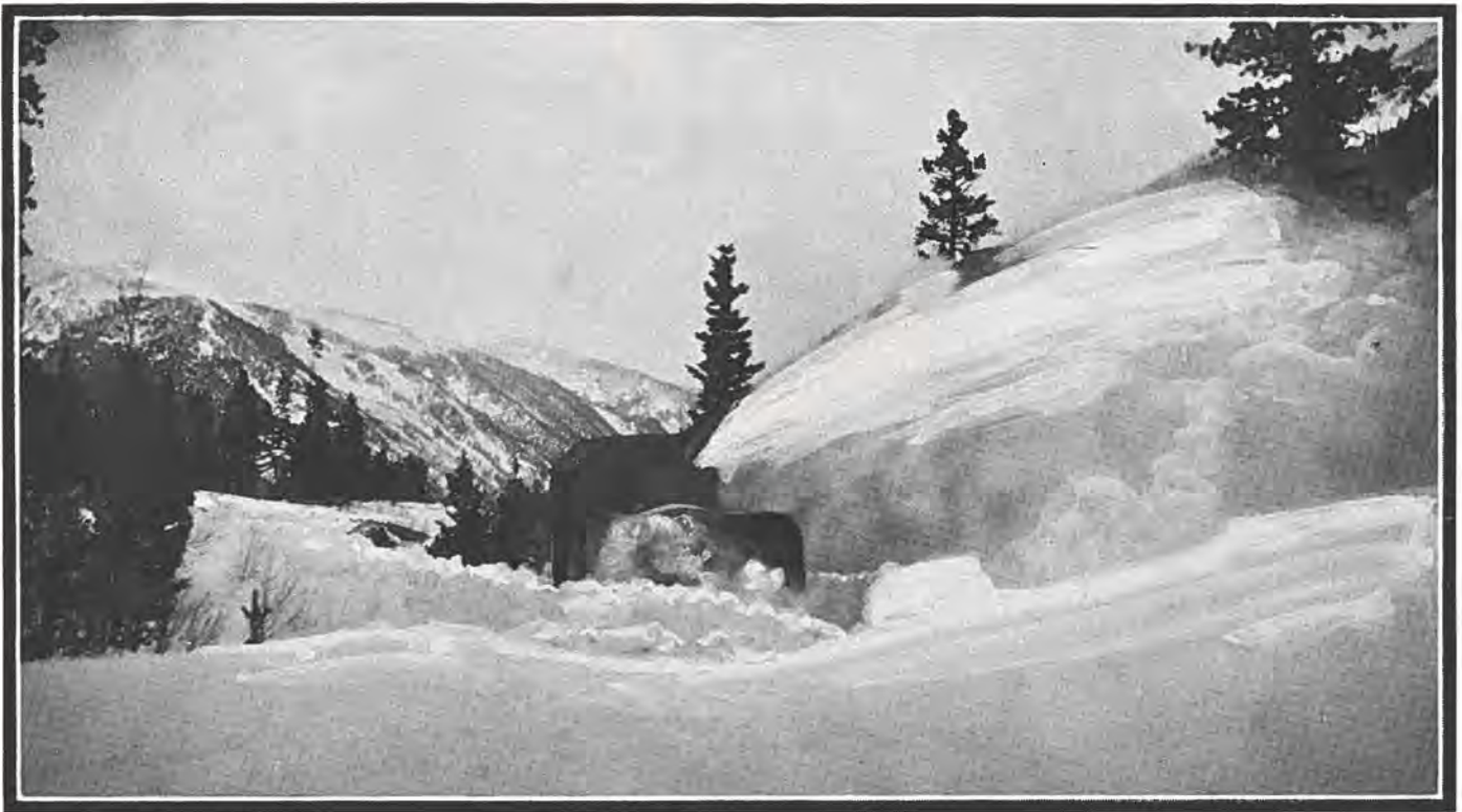
Giant State Highway Department rotary snow plow working on Berthoud Pass.
