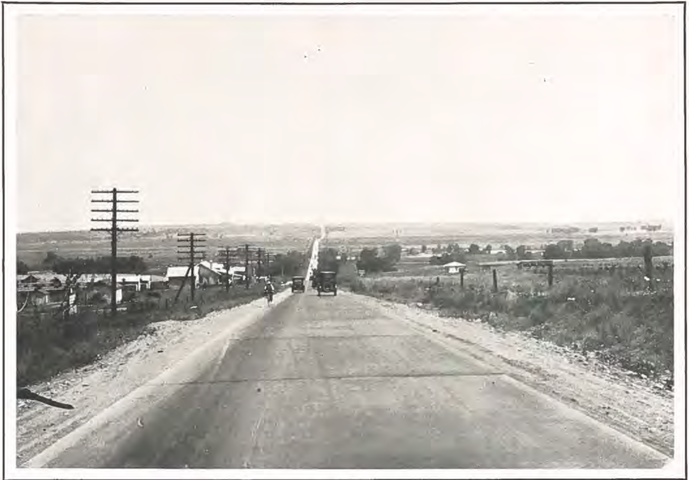
One of the main routes serving Northern Colorado—the concrete paved Lincoln Highway in Adams County.
