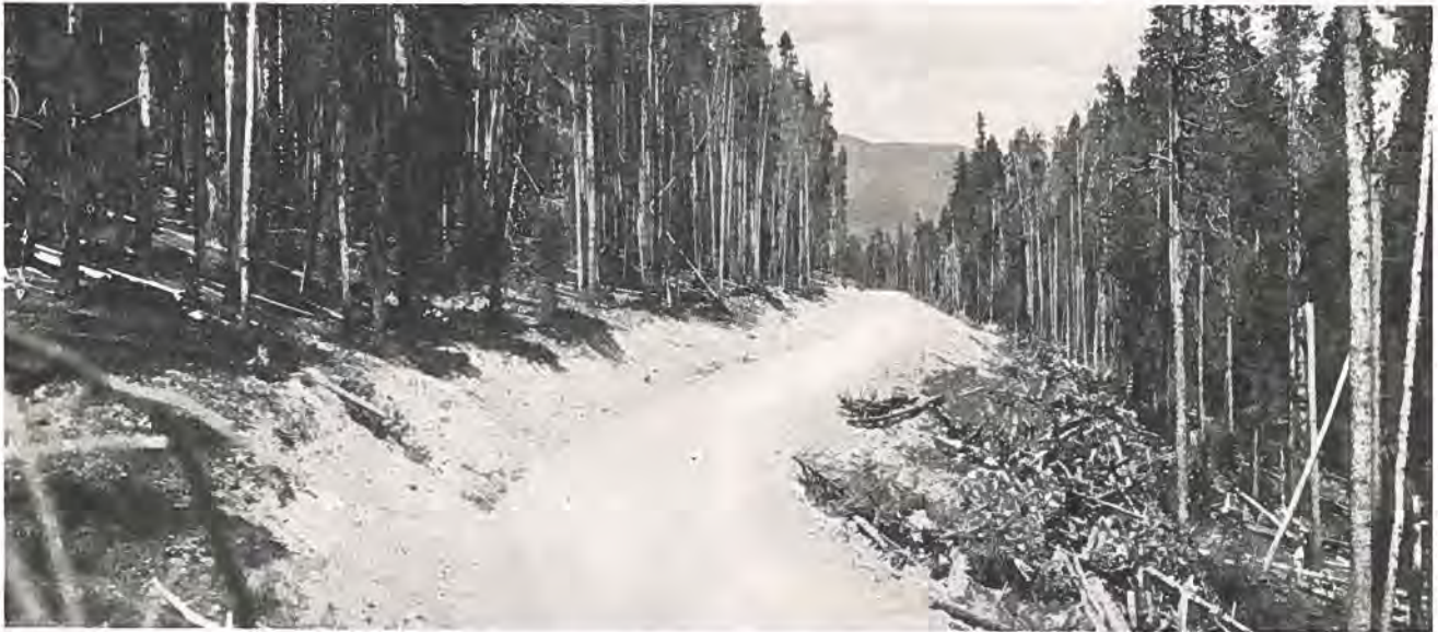
Showing a stretch of gravel surfaced highway on Willow Creek Pass recently completed by the U. S. Bureau of Public Roads. It is located in the Arapahoe National Forest and the new road eliminates the worst stretch between Granby and Walden.
