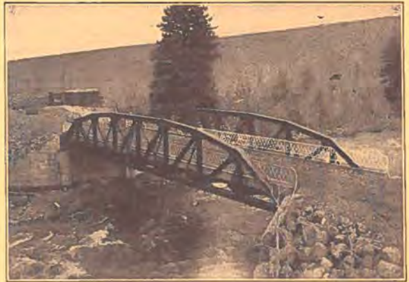
100 ft. Riveted Low Truss Span, Dillon, Colo.
