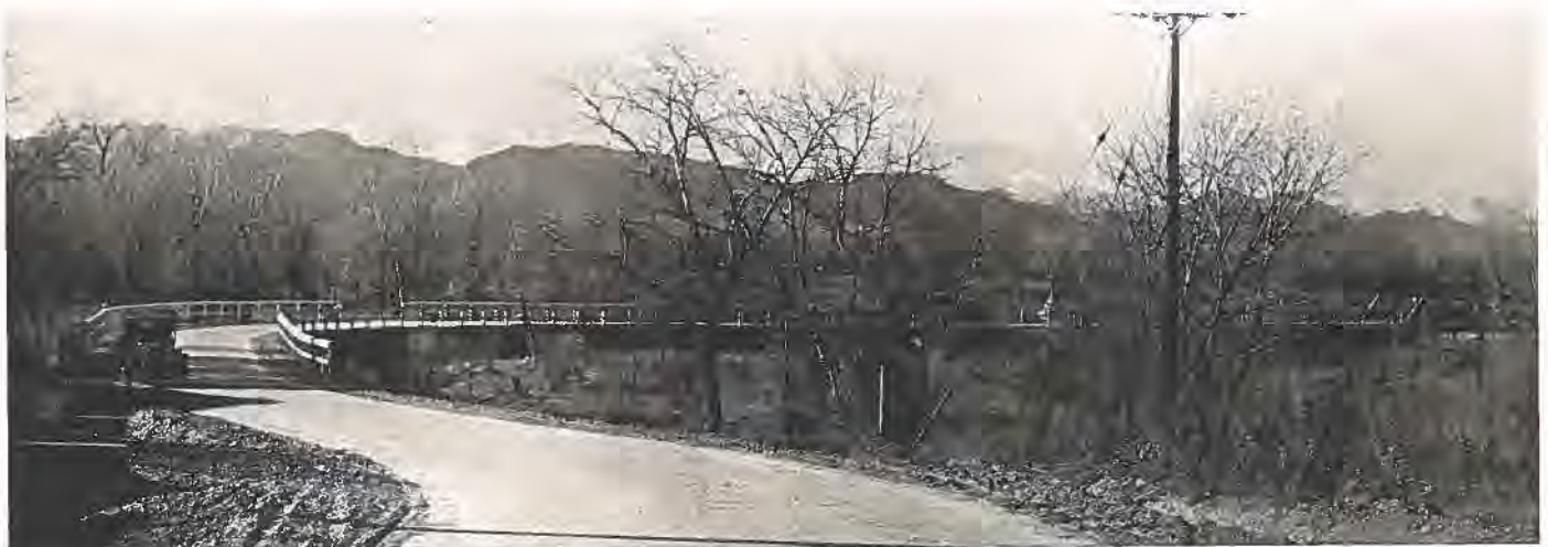
Where an artist would stand enthralled. The scene is on the state highway built by the Highway Department between Denver and Arvada. Here is the concrete road, the bridge across Clear Creek, with its foliage-covered banks, and in the background the foothills and the snow-covered Continental Divide beyond.
