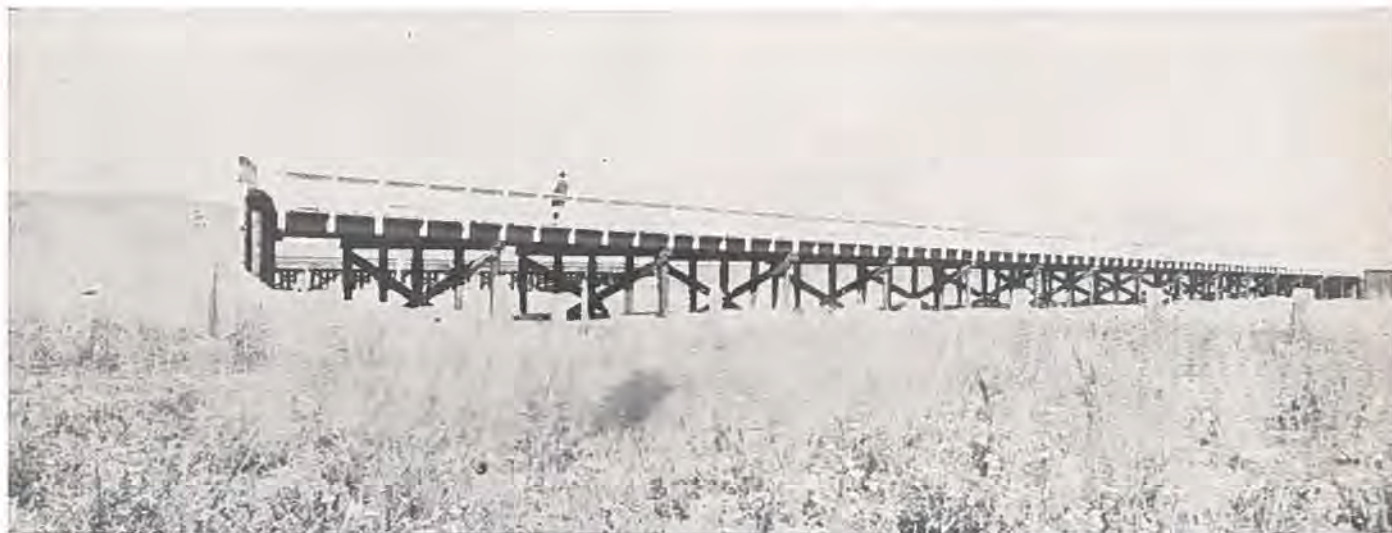
Treated timber pile bridge located east of Bennett on Denver-Limon highway, constructed with Federal Aid funds.
