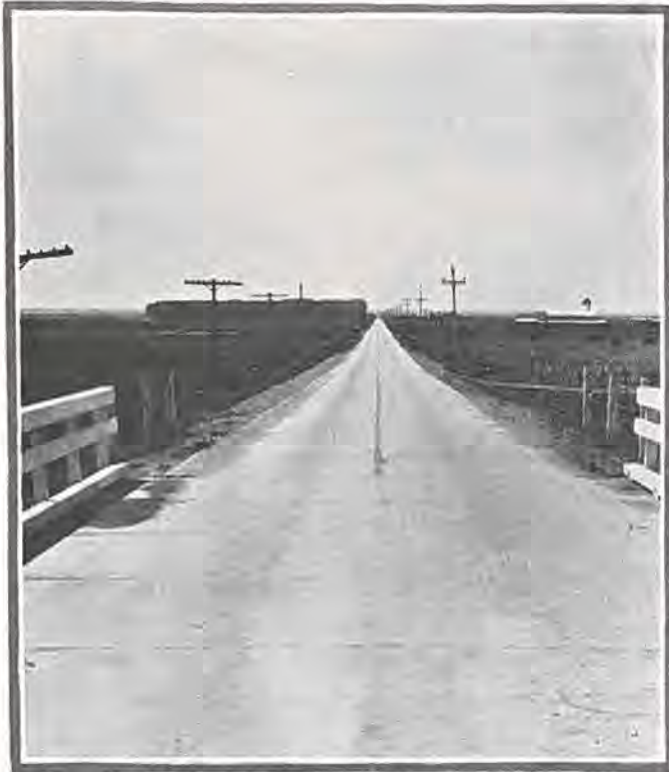
Showing completed concrete pavement between Sterling and Fort Morgan.
