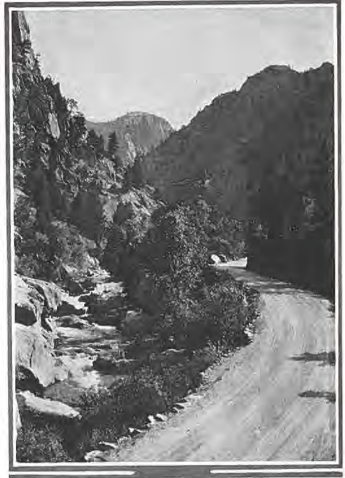
Stretch of new road in South St. Vrain Canon.
