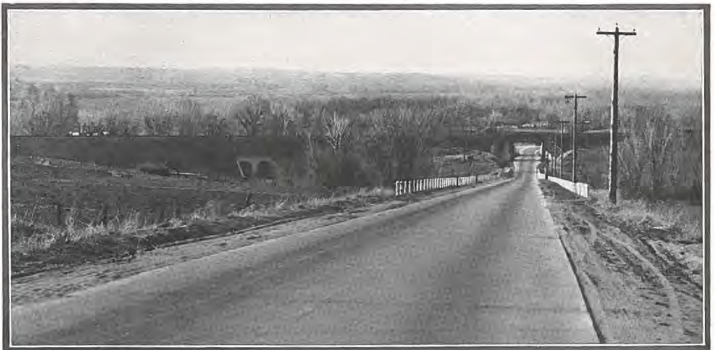
A stretch of concrete pavement on the Colorado Springs-Denver concrete boulevard, showing one of the many underpasses eliminating railroad grade crossings.
