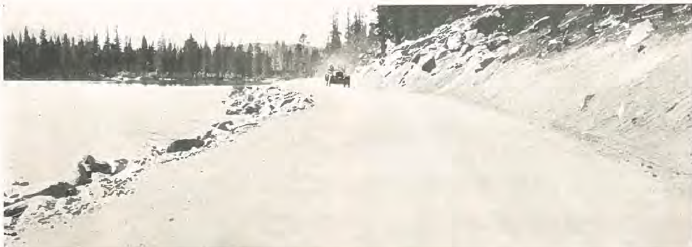
A section of the Echo Lake-Idaho Springs highway, showing the smooth and wide gravelled surface, with the lake at the left.
