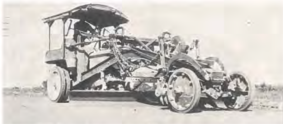
Galion one-man grader being operated by State Highway Department between Pueblo and Colorado Springs. This outfit travels an average of 23 miles a day.
