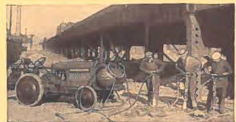
Air-compressor outfit powered by a McCormick-Deering tractor, used by a Philadelphia contractor.
