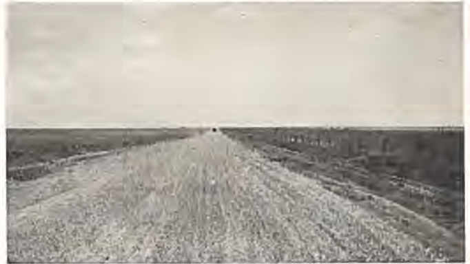
A glimpse of the finished oiled road between Nunn and the Wyoming state line, State Highway No. 3. Motorists are loud in their praise of this new type of surfacing.—Photographs by Roy J. Randall.
