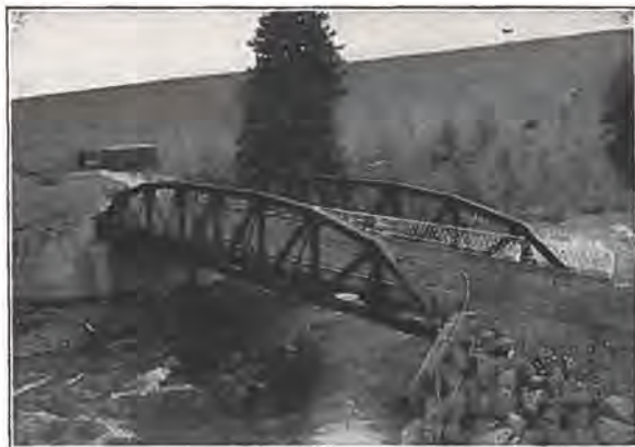
100 ft. Riveted Low Truss Span, Dillon, Colo.
