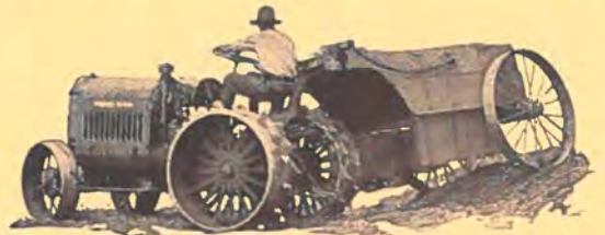
Last January, at the Cleveland Road Show, 24 exhibitors showed 48 McCormick Deering tractors. Each year has shown a tremendous increase. Regarding the outfit shown above, the superintendent of construction, Minnesota Trunk Highway No. 20, writes: "I never thought it possible to move dirt so cheaply and so quickly."
