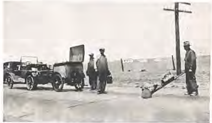
A state maintenance crew filling expansion joints on concrete pavement.
