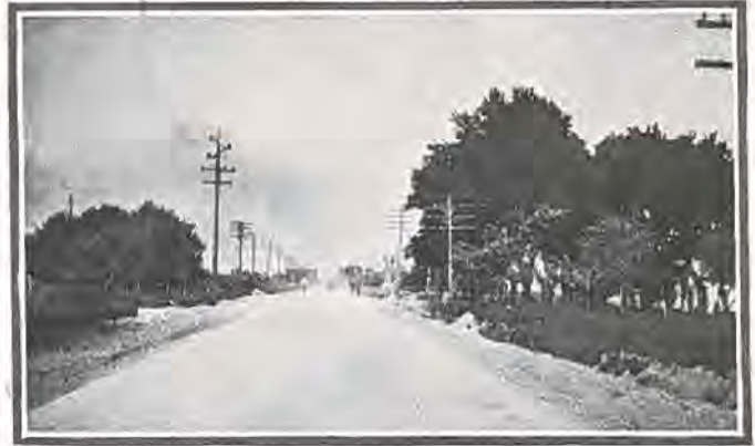
Section of concrete pavement east of Grand Junction, leading into the Palisade fruit section.
