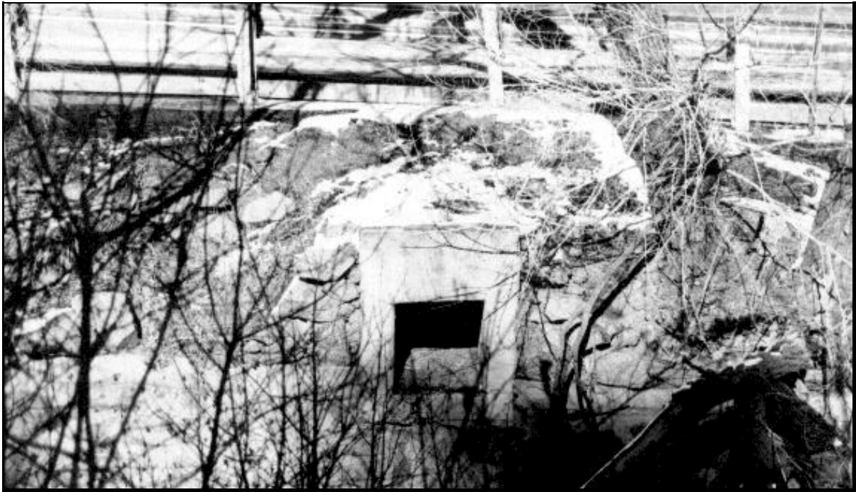
Plate 34. Concrete culvert inside rock work. View from east side of US 24.
