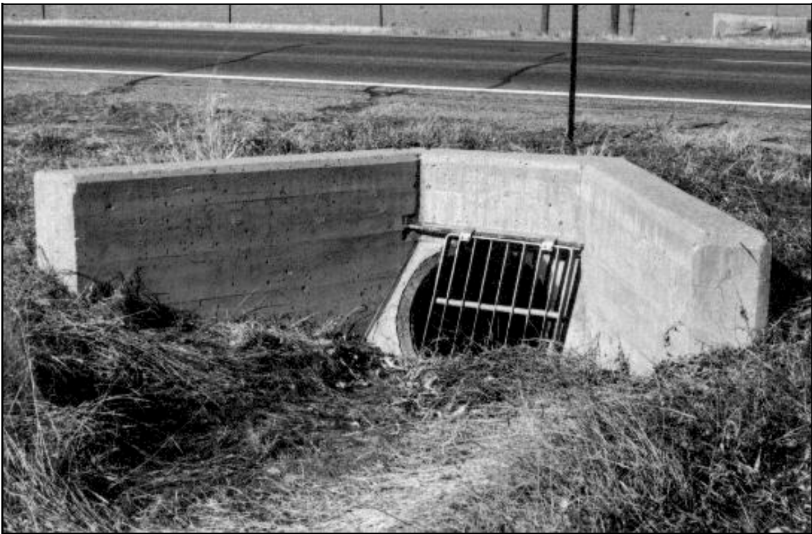
Plate 21. Concrete culvert with grate. North of Merino on US 6.
