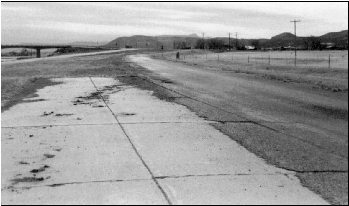
Plate 25. Old asphalt gives way to concrete. Southwest view of US 85.
