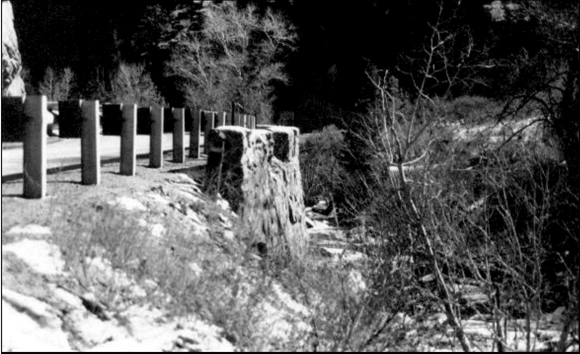
Plate 36. Cement and masonry wall from inside the guardrail above Fountain Creek.
