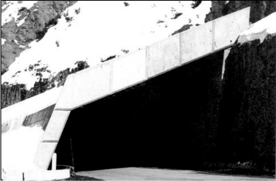
Plate 11. Northeast view of Riverside Slide, a block and concrete tunnel.
