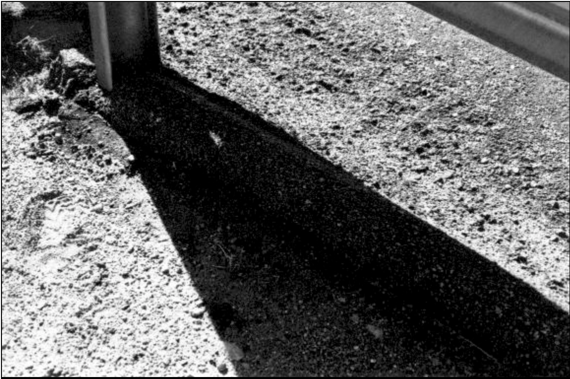
Plate 22. Asphalt mountable curbing inside guardrail on US 6.
