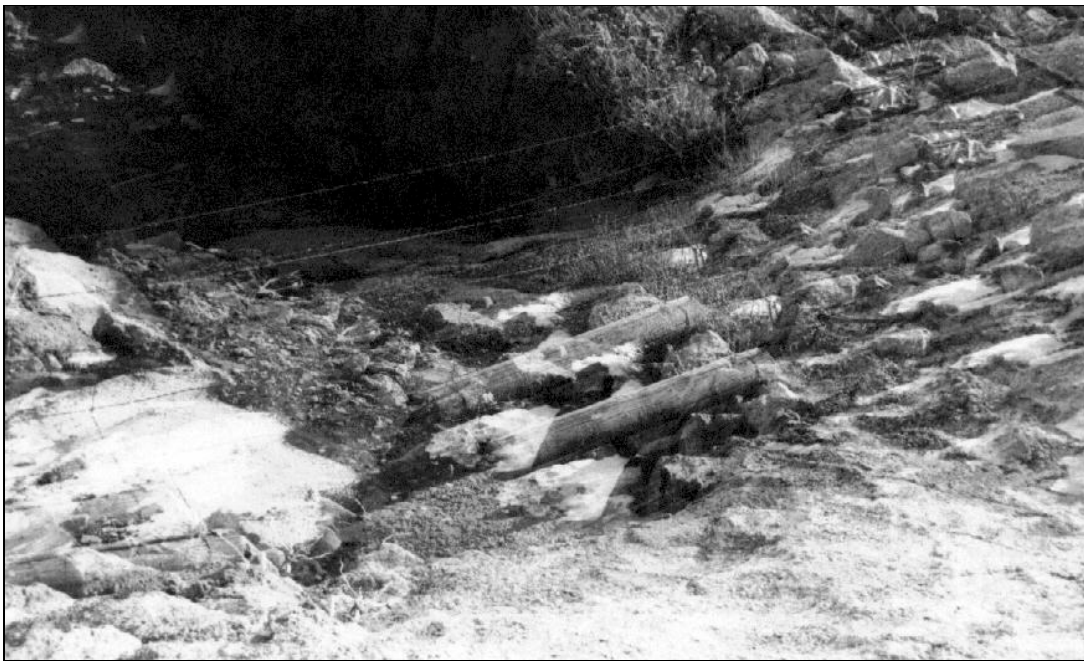
Plate 27. West view of wooden culvert on old US 85, Las Animas County.
