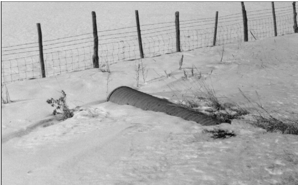
Plate 32. Corrugated metal culvert viewed from the west side of SH 13.
