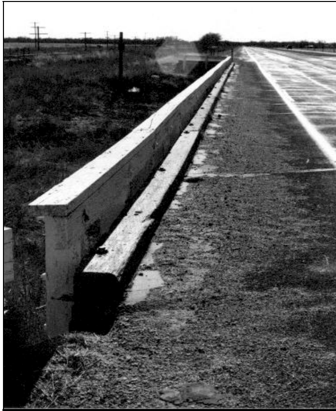
Plate 18. Timber curbing along bridge over Pawnee Creek, Logan County. View south down US 6.
