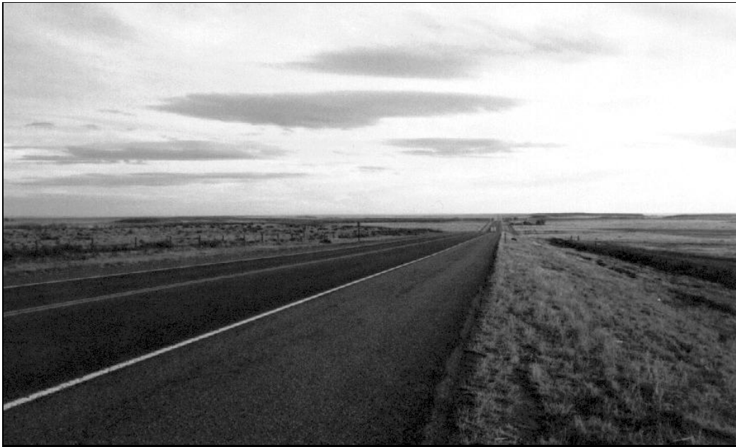
Plate 28. Steep embankments on both sides of US 385 southwest of Lamar near the local airport.
