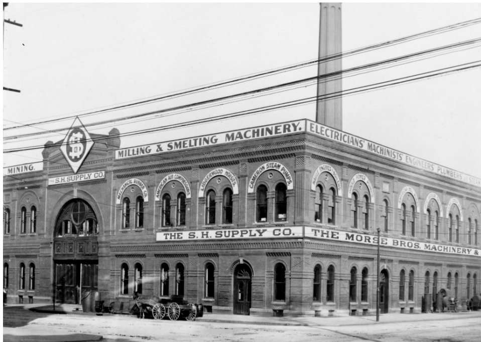
Figure 189. The extant Denver City Cable Railway Company power plant, 1906. 765
