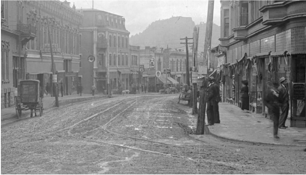
Figure 177. Photo of streetcar tracks on Commercial Street, looking north from Main Street, c.1890-1900. 750
