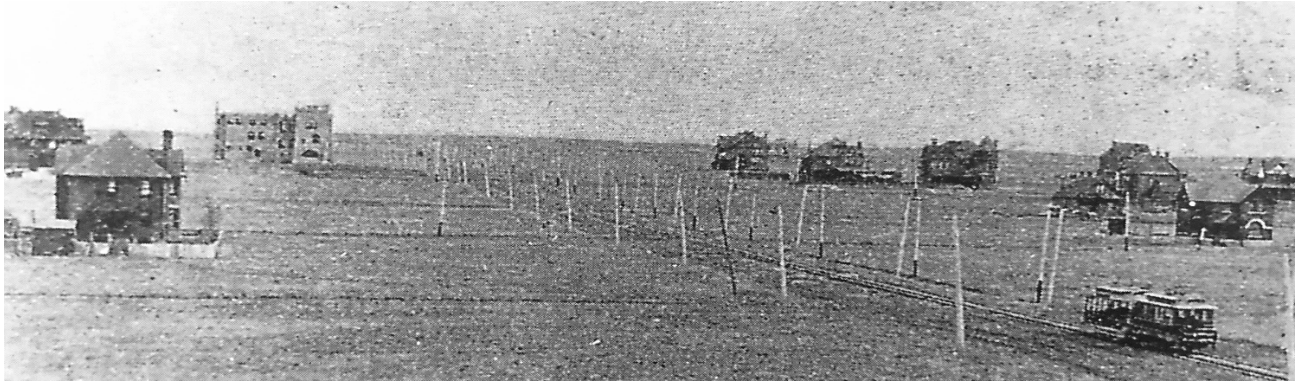
Figure 82. View of the Montclair Railroad Company line along East 8 th Avenue, looking west from Quebec Street. 424
