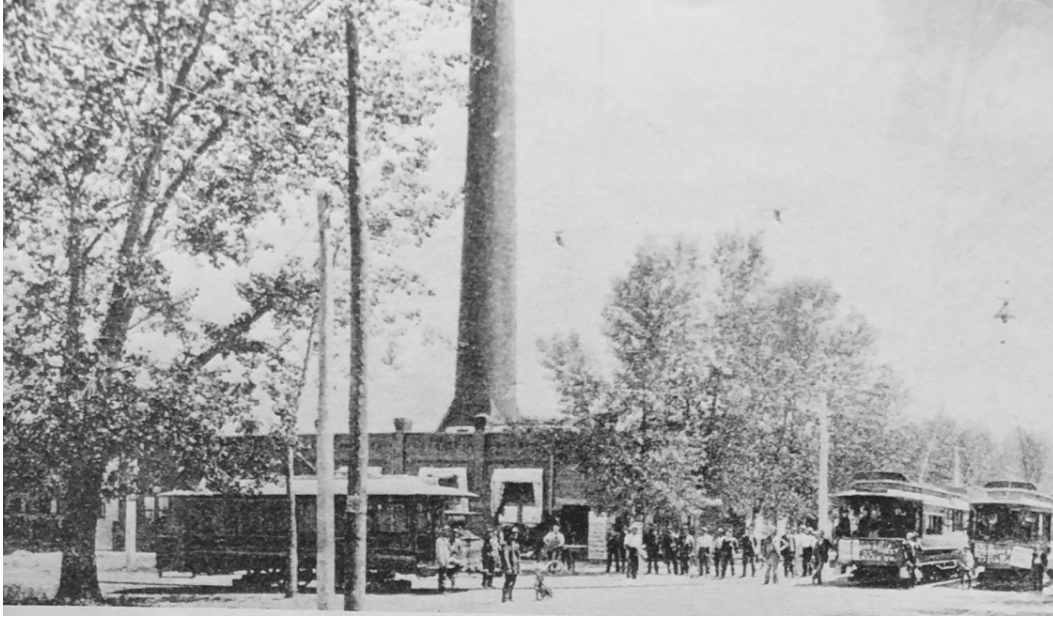
Figure 88. WESR cars in front of their powerhouse and carbarn at West 38 th Avenue and Utica Street. 454
