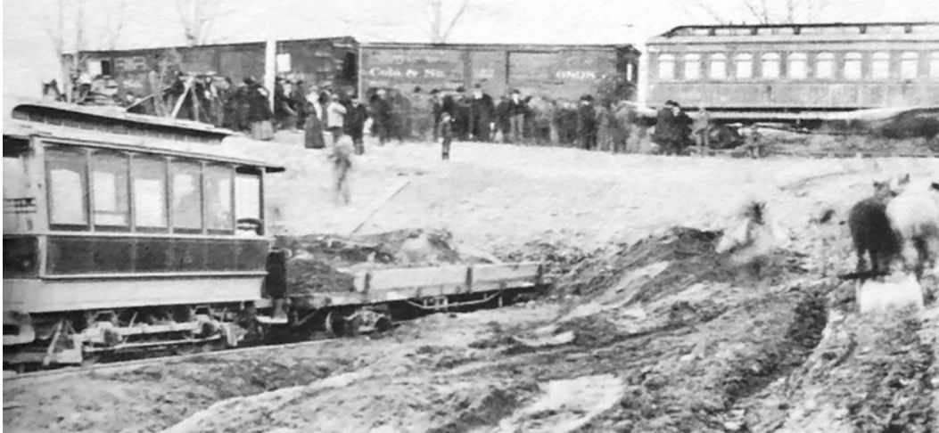
Figure 104. Site of D&NW crossing with the C&S, under construction, 1902. 509
