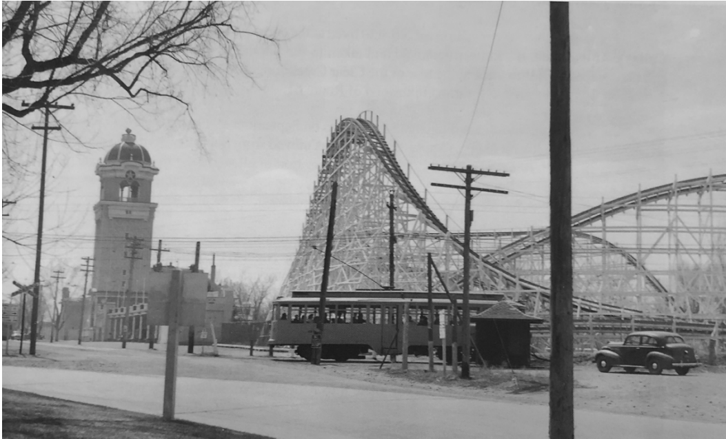
Figure 110. Interurban car from D&NW route passing Lakeside Amusement Park at West 48 th Avenue and Sheridan Boulevard. 526
