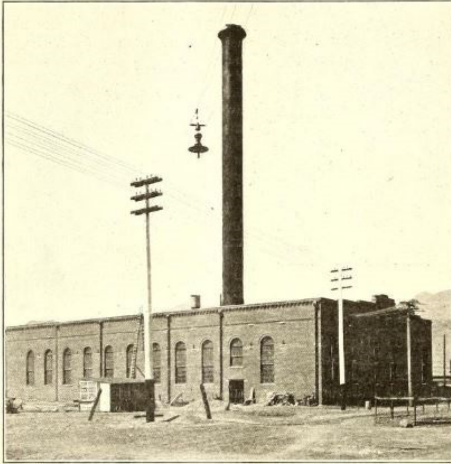
Figure 34. Power plant constructed by the CS&I at Sierra Madre Street and Rio Grande Street, 1902. 222
