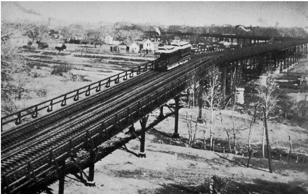
Figure 54. View of west end of Larimer Street Viaduct with a DCCRC car on it. 282
