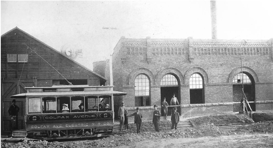
Figure 80. CAERR in front of their powerhouse at East Colfax Avenue and Ulster Street when it was under construction, c.1890. 406
