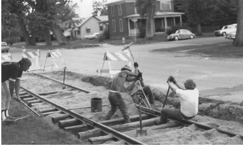
Figure 142. Volunteers complete the reconstruction of the Mountain Avenue line, 1986. 643
