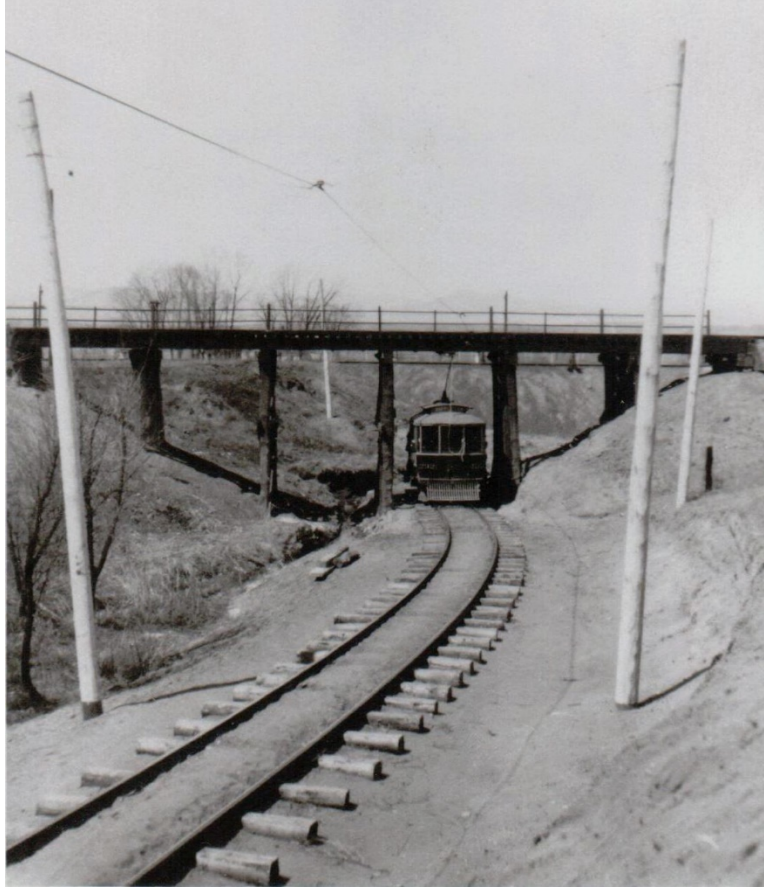
Figure 164. D&SP streetcar in Slaughterhouse Gulch, c.1910. Note the poles carrying the electric lines installed at an angle outward to keep the electric lines taut. 710 (Image from the Collection of the Littleton Museum. May not be reproduced in any form without permission of the Littleton Museum.)
