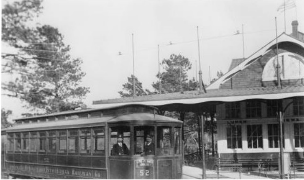
Figure 36. Streetcar and car pavilion at Stratton Park, c.1901-1910. 225
