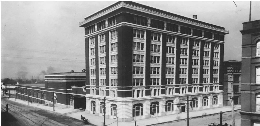
Figure 64. New Tramway central office building at 14 th and Arapahoe Streets with attached Central Division Car House, 1911. 333
