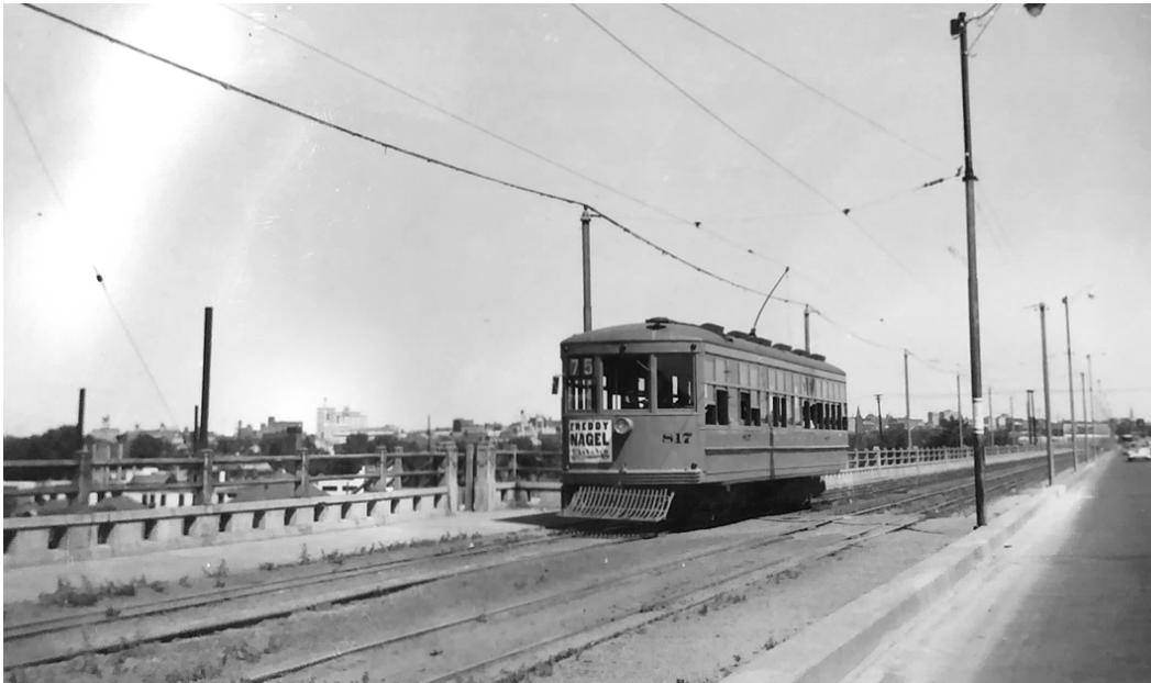
Figure 67. Car on West Colfax Viaduct, 1943. 342
