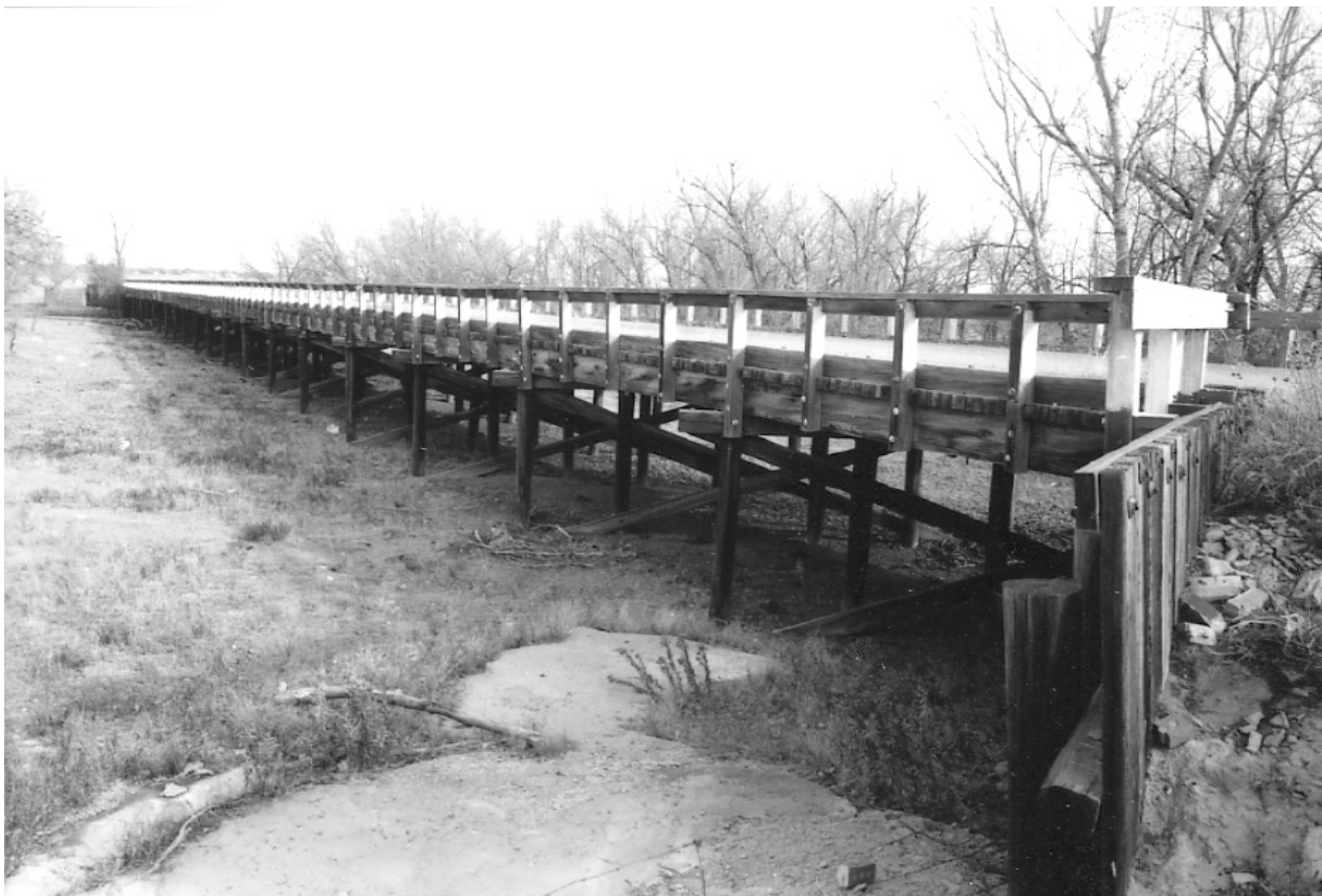
Big Sandy Creek Bridge 5CH157-2
