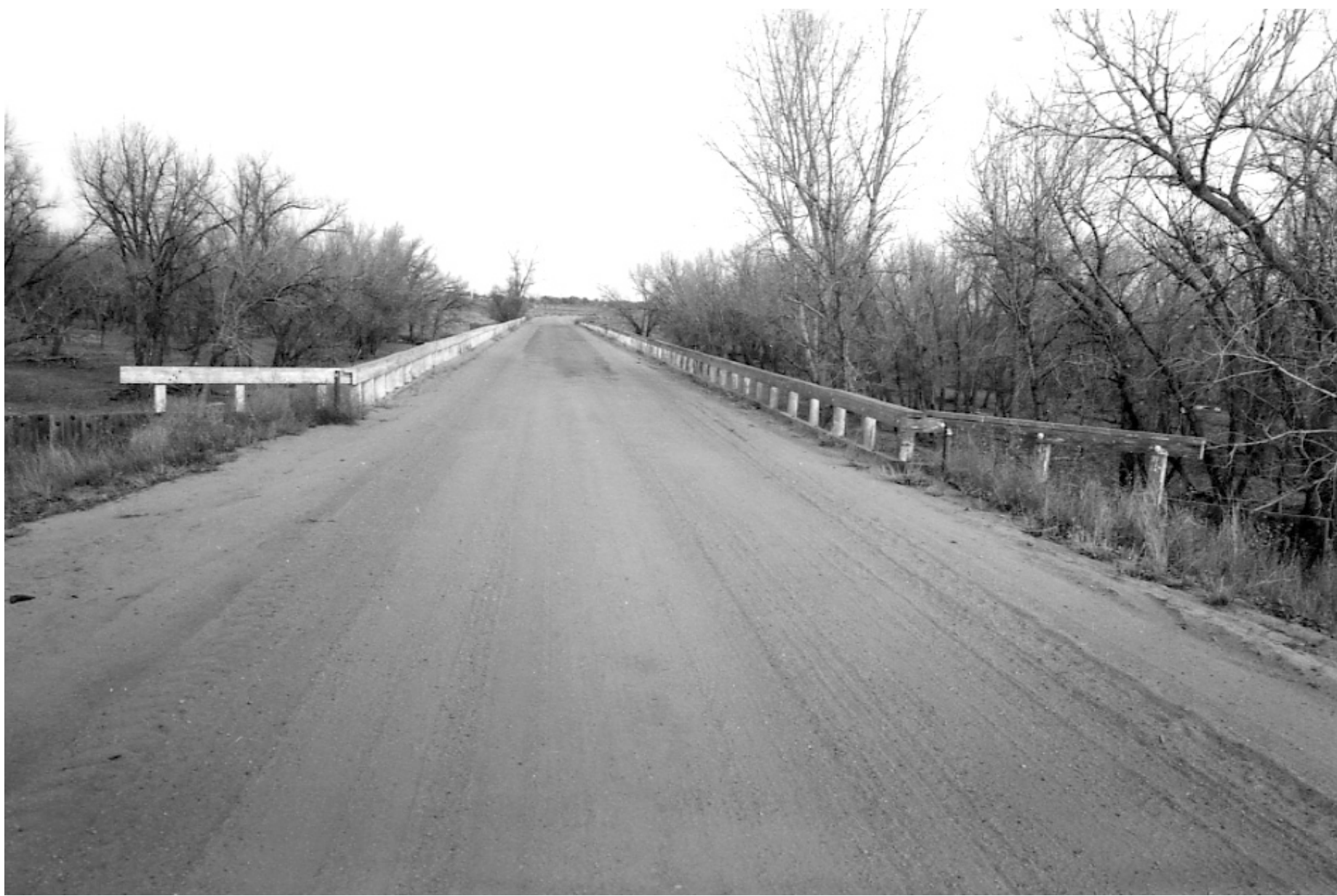
Big Sandy Creek Bridge 5CH157-1
