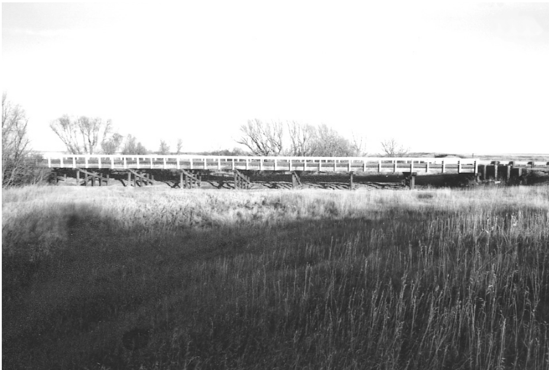
Sandy Creek Bridge 5PL40-2
