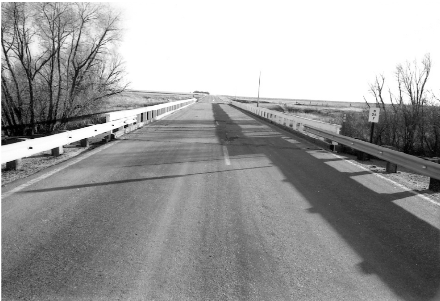
Sandy Creek Bridge 5PL40-1
