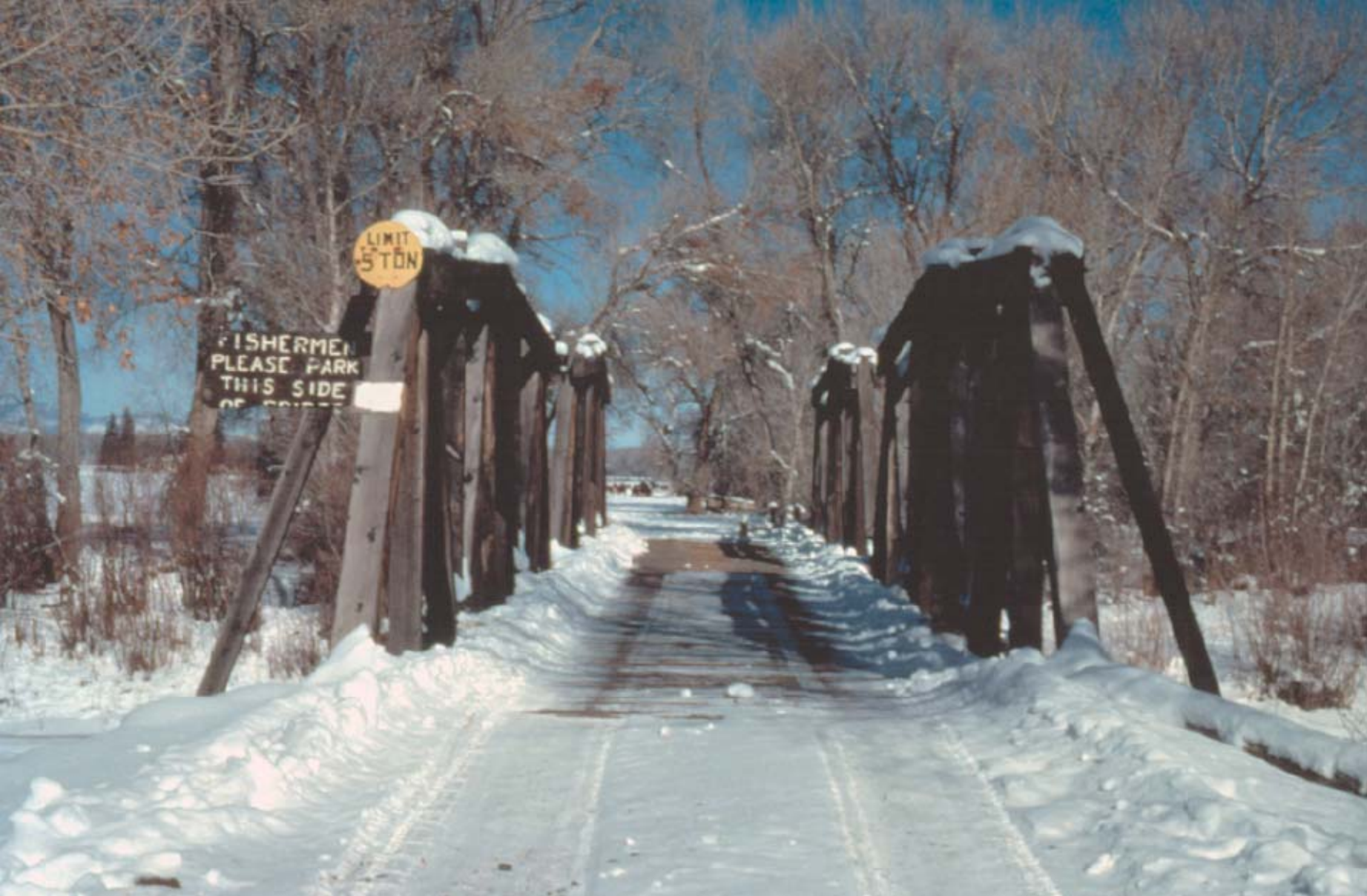
Wheeler Bridge 5RN400-1(C)
