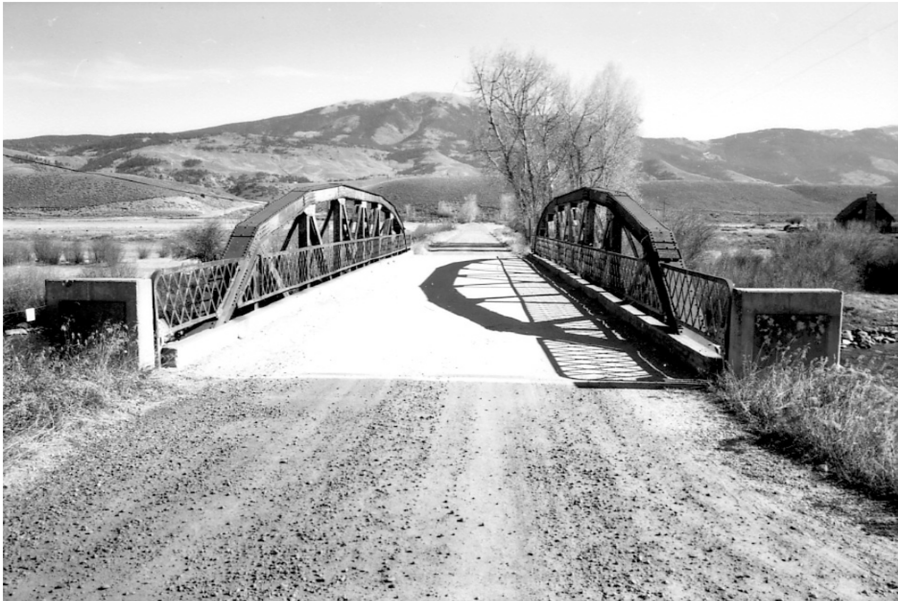
Slate Creek Bridge 5ST324-1
