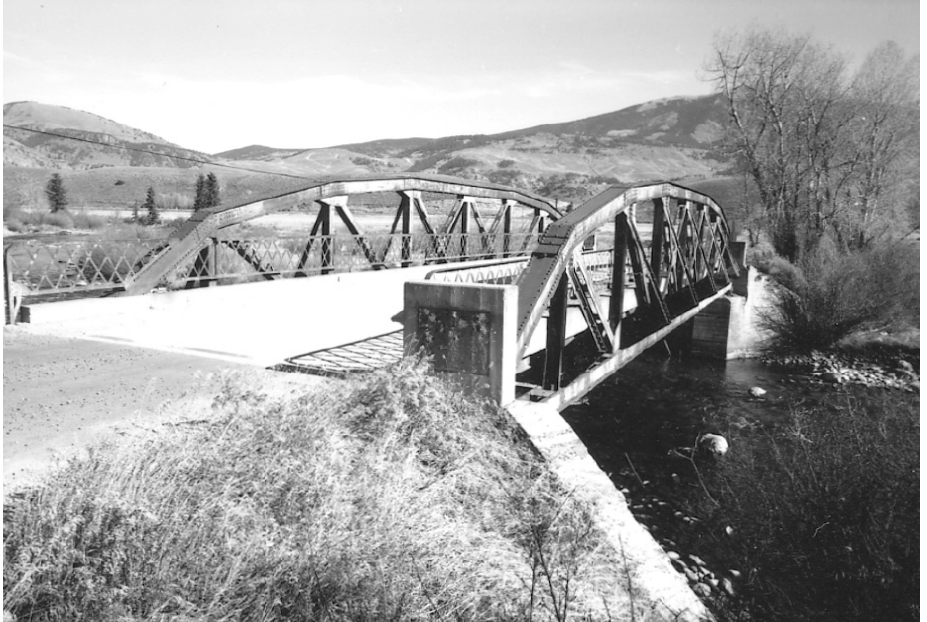
Slate Creek Bridge 5ST324-2
