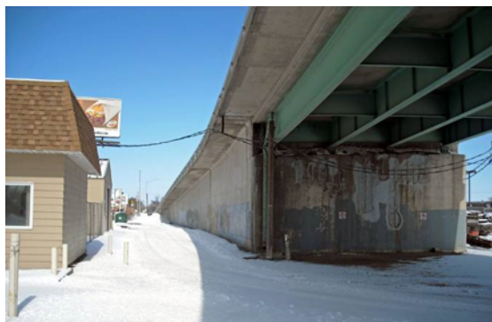
Paint on old bridges may contain heavy metal-based paint.
