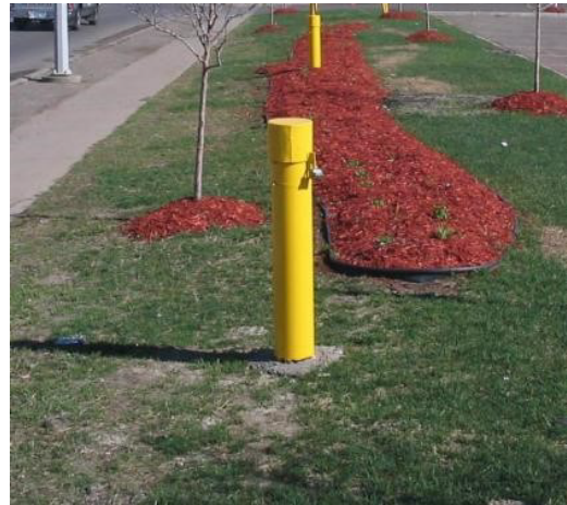
Figure 4.25. Above-Grade Completion of a Groundwater Monitoring Well
