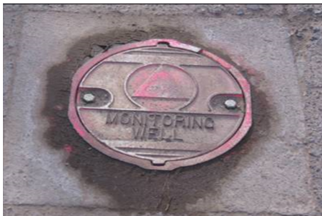
Typical in-ground monitoring well.
