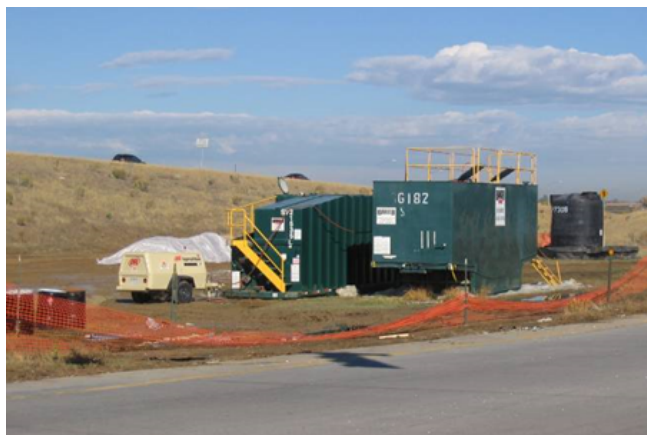
Baker remediation tank in highway right-of-way.
