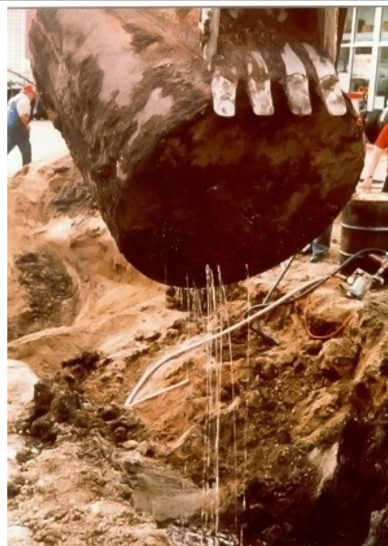
Figure 4.22. Steel Underground Storage Tank Leaking During Excavation
