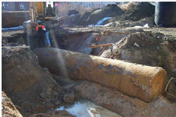
Figure 4.21. Steel Underground Storage Tank Being Excavated
