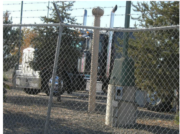
Vent pipe that may be connected to a former landfill beneath the ground surface.
