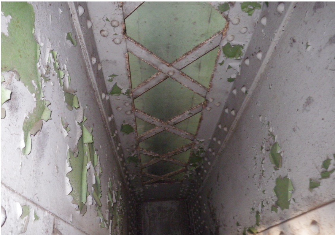
Figure 4.17. Heavy Metal-Based Paint Chipping
