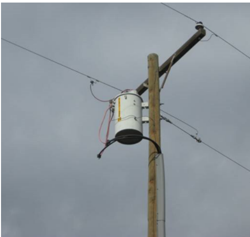
Pole-mounted electrical transformer in highway right-of-way.
