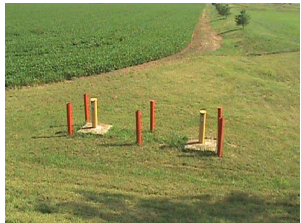
Monitoring wells in a non-commercial setting.
