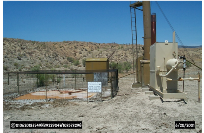
Produced water pit at a natural gas well.
