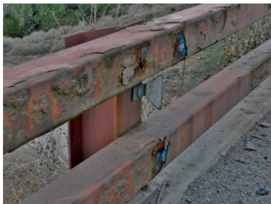
Chipping paint on a bridge rail may contain heavy metal-based paint
