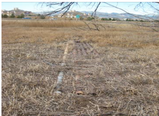
Old pipes adjacent to the highway right-of-way.
