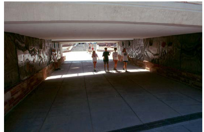
Figure 4.h: Good lighting enhances this well placed pedestrian underpass that connects existing pedestrian circulation networks.
