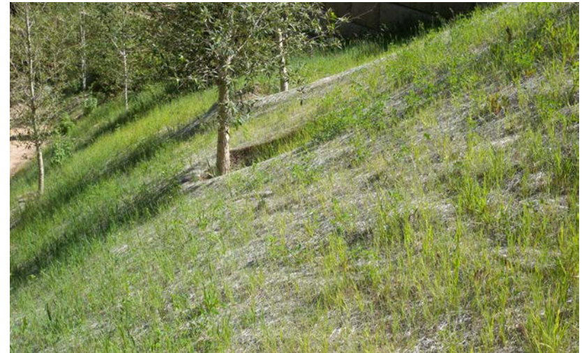
Figure 2.w: A variety of techniques are used in this urban setting. They include chain link fencing for site protection, straw erosion control matting and black silt fencing to trap sediments.
