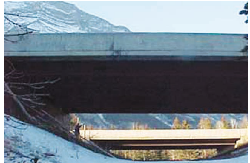
Figure 2.f: This raised roadway crossing over a natural drainage provides a wildlife movement corridor.
