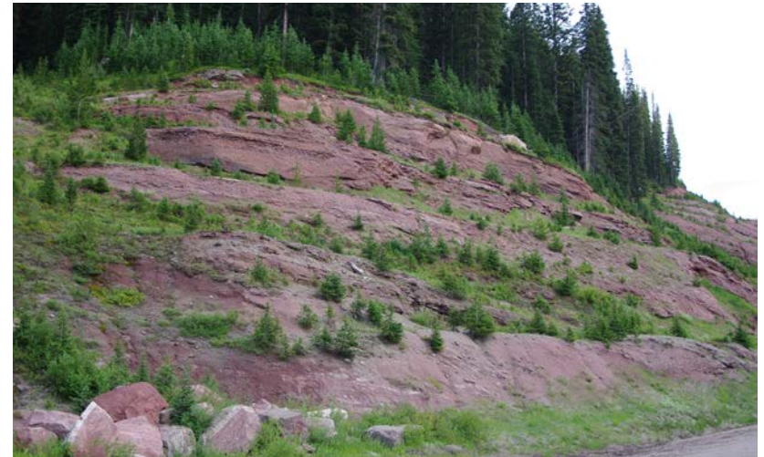
Figure 2.r: Naturalized cuts and benches, as in this example, are encouraged.
