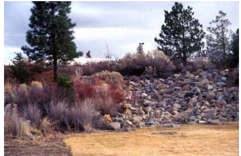
Figure 2.ze: Rock riprap is integrated into a vegetated slope.
