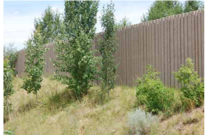
Figure 3.zb: The use of grading allows for reduction in height of the wall and also for landscape planting.
