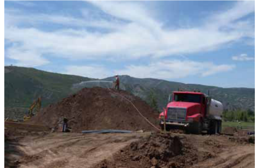
Figure 2.zzh: Topsoil is stockpiled on site and watered to minimize dust.
