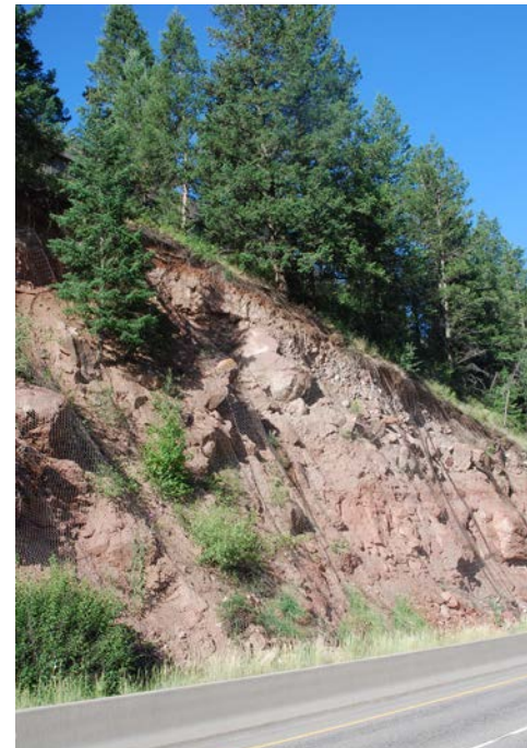
Figure 2.s: Soil nail techniques are used for stabilizing rock faces.
