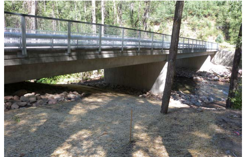
Figure 2.u: A combination of river rock rip rap and reseeded protected by erosion control blankets are used in the streambanks. These are examples of heights steps, transitions and ends. The top left angular, irregular pattern should be avoided.
