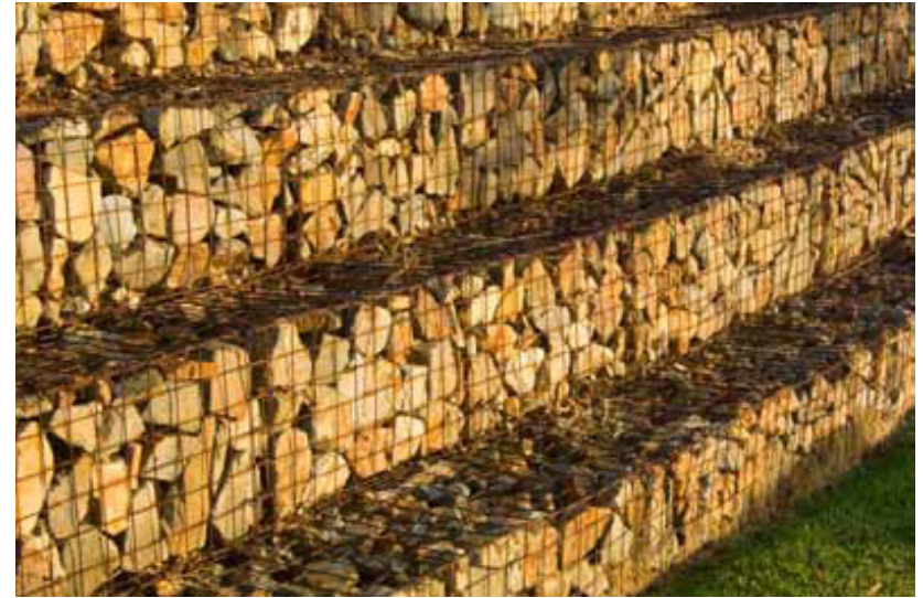
Figure 2.zf: Well constructed rock gabions.
