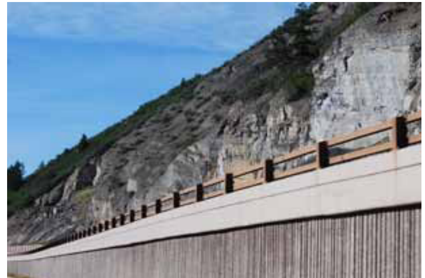
Figure 3.zi: Barriers with vertical fluted treatments enhance light and shadow effects.
