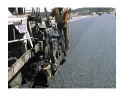
placement of asphalt rubber. To ensure the highest quality, the placement temperatures must be 65 degrees and rising. This makes night paving in Colorado virtually impossible. Since traffic congestion requires most construction in Colorado, especially in urban areas such as Denver and Colorado Springs, to be conducted at night, there is a very small window of opportunity to pave.
