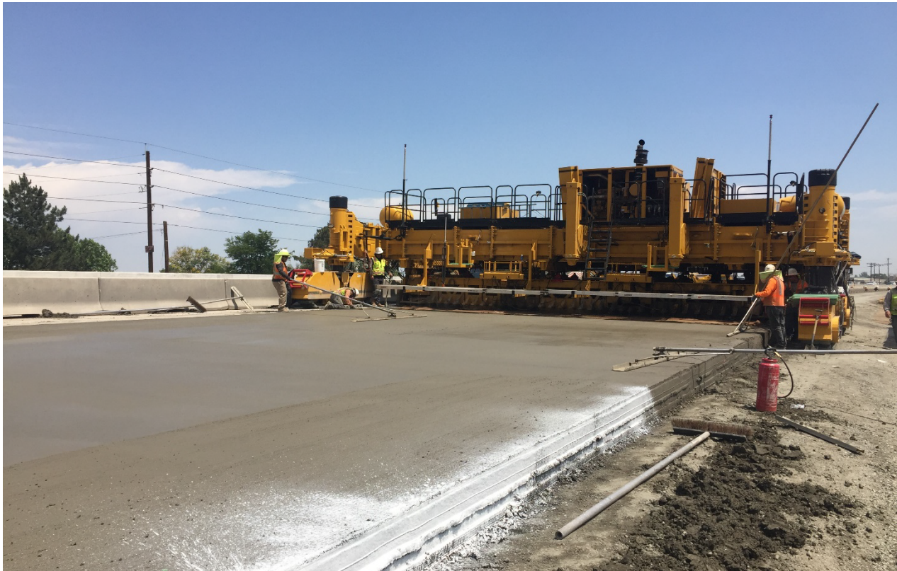
Figure 4.12. New Highway Under Construction
