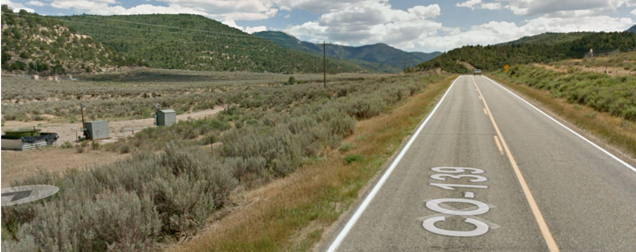
A gas well located adjacent to highway right-of-way on the left of the highway; an unmarked collection pipeline on the right of the highway.
