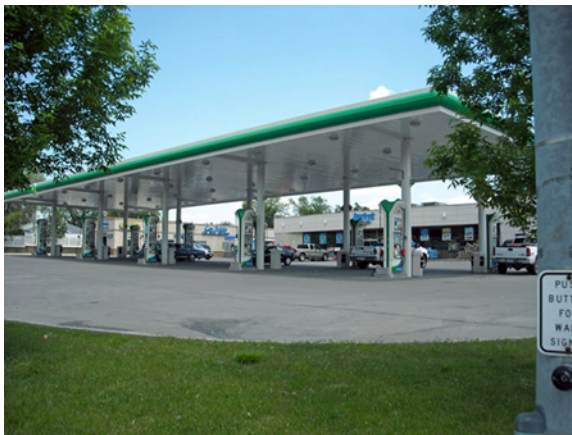
Typical modern filling station.
