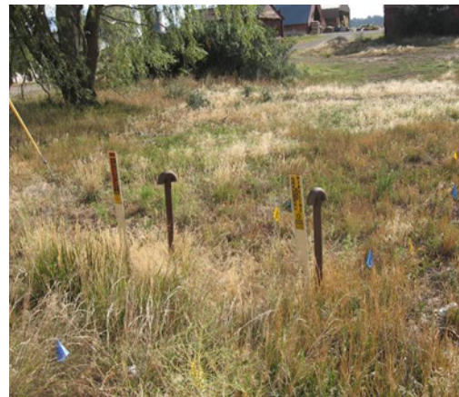
Gas pipeline vent pipes adjacent to highway right-of-way.
