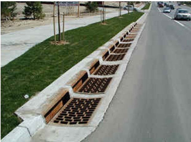
A set of storm sewer inlets along a roadway.
