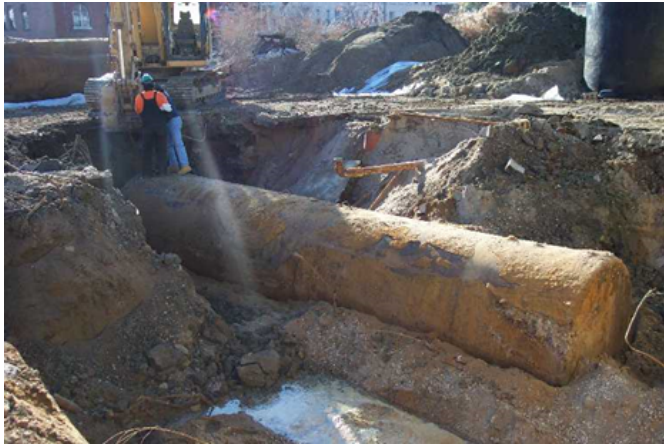
Figure 4.21. Steel Underground Storage Tank Being Excavated
