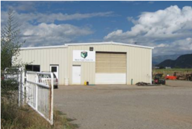
Two 55-gallon drums (to the right of the garage) associated with property adjacent to highway right-of-way. One drum is tipped over.
