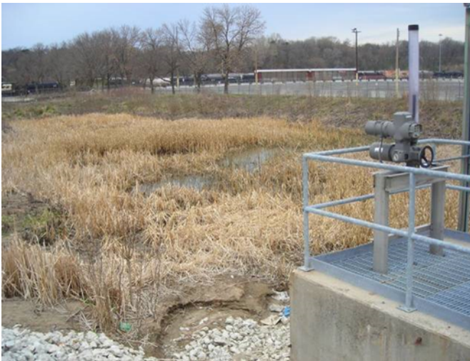
Detention pond at an agricultural chemical manufacturing facility.
