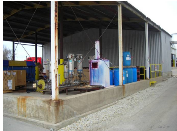
Covered hazardous materials storage area with secondary containment.
