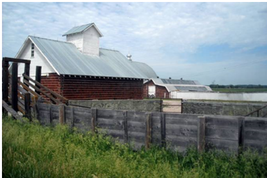
Paint on old buildings may contain heavy metal-based paint.
