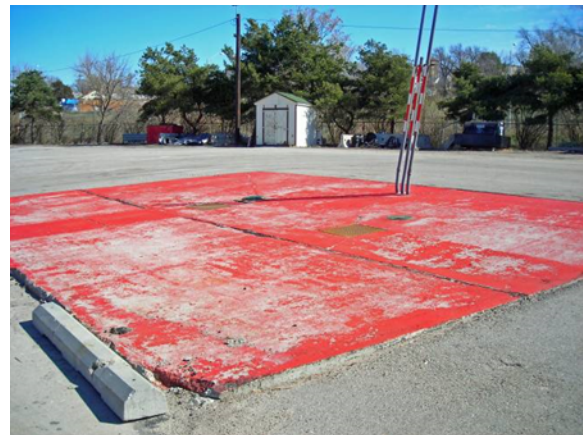
Fill caps and vents in a concrete surface.
