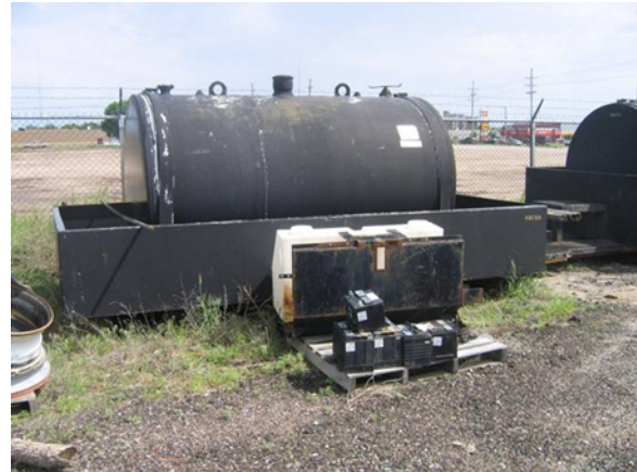
Old batteries stored outside and exposed to the elements. Also, AST with secondary containment.
