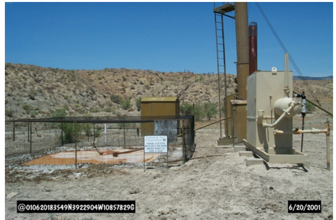
Produced water pit at a natural gas well.
