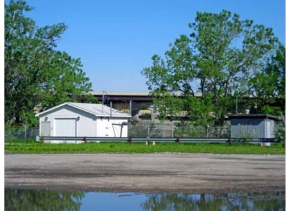
Typical groundwater remediation sheds.
