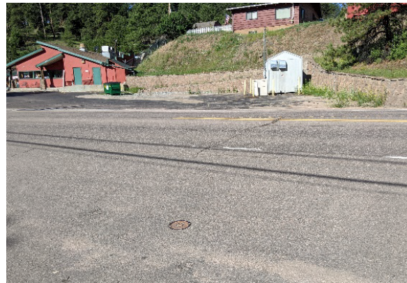
Groundwater remediation shed in the background with a monitoring well in the foreground
