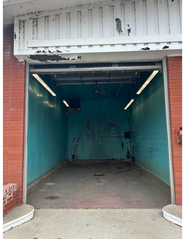
Evidence of a former vehicle maintenance bay and former hydraulic lift.
