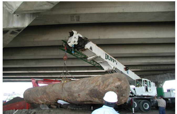
UST removal associated with a transportation project.
