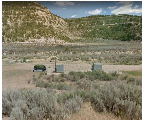
AST at a natural gas well adjacent to the highway.
