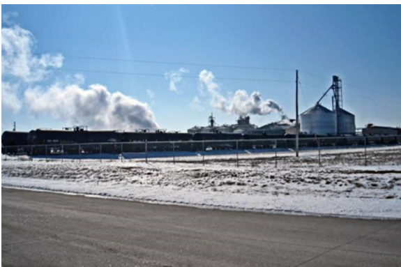
Railroad access line for an ethanol plant.
