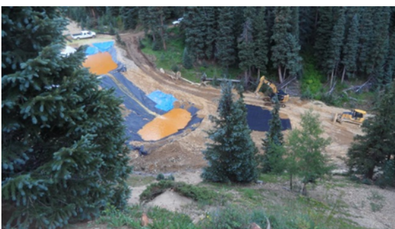
Emergency tailing ponds constructed in response to a spill.
