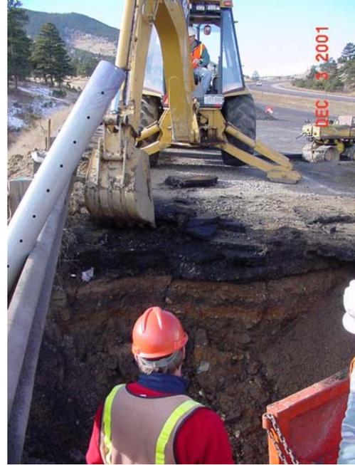
Figure 2.3 Mitigating groundwater problems.
