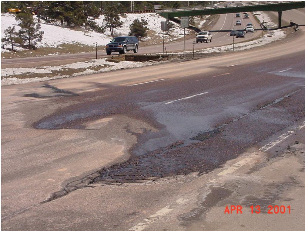
Figure 2.1 Groundwater problem in a highway (I-70 at Floyd Hill).
