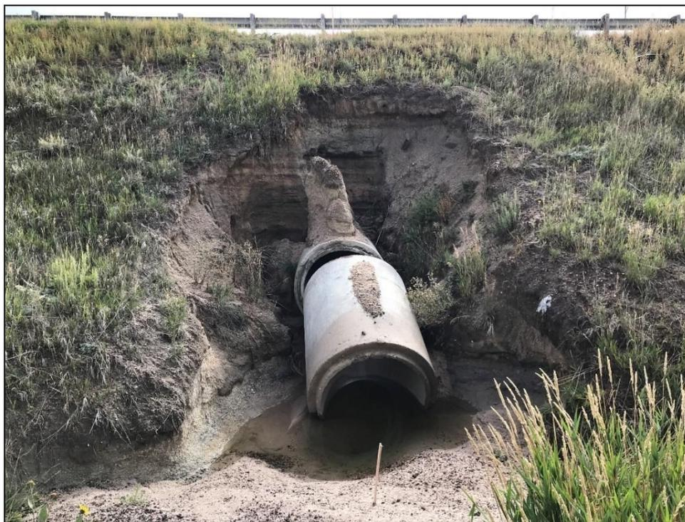
**Photo 11.1** Culvert outlet failure on I 25 near milepoint 162.1, 9/6/2018
