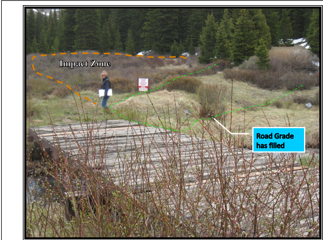
Figure 42. Wetland off of CO Hwy. 9. Fill was placed across a portion of the wetland to form a road grade. Affected areas are no longer wetland. If the AA was delineated according to the wetland boundary, this geomorphic impact would be excluded and not be taken into account in Geomorphology Variable scoring. The effects of the fill on functioning in the AA would be documented when scoring other variables, such as Water Distribution (see illustration at left). This approach would commonly be taken during the project permitting when the focus is specifically on determining impacts to regulated habitats.
