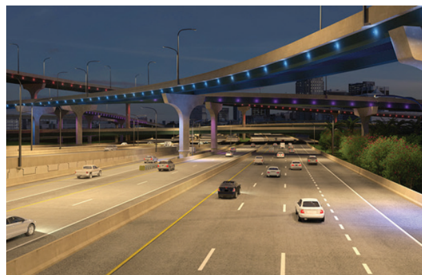
I-4 Ultimate Project - Project 1
