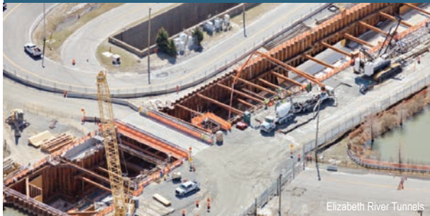
Elizabeth River Tunnels
