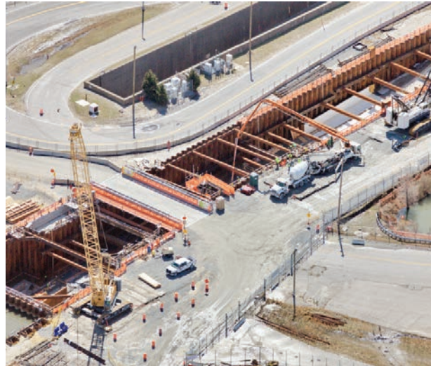
Elizabeth River Tunnels
