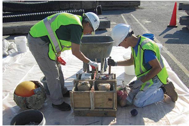
Our Elizabeth River Tunnels team is using waste concrete to make oyster boxes for the Elizabeth River.
