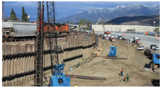
Skanska utilized heavy shoring for highway construction near an operating railroad during I-215 construction in San Bernardino, CA
