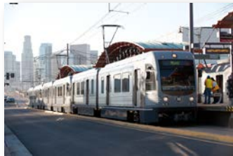
The Eastside Extension Project was the first Metro project to be delivered via a design-build delivery method.
