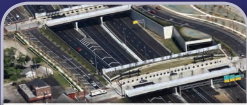
Phased Deep Excavation I-71/670 Columbus Crossroads
