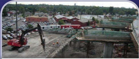
Viaduct Removal (demolition) Broadway Demo
