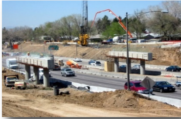
The Steele Street Bridge design and construction required detailed planning an execution of the works to keep the workers and traveling public safe during the construction adjacent to live traffic.
