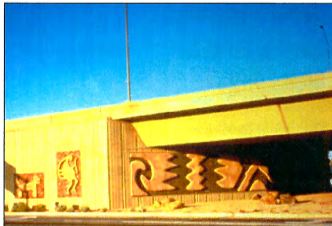
Sample of Phoenix art work at bridge retaining wall.
