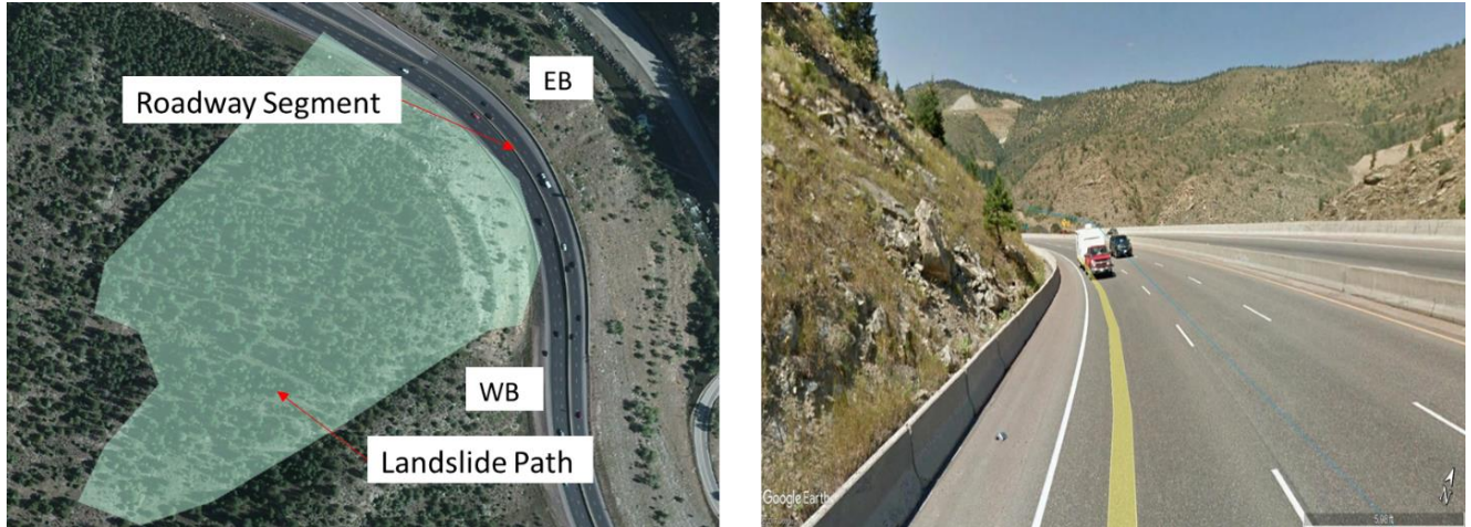
Figure 18. Site 3 near MP 244.5
