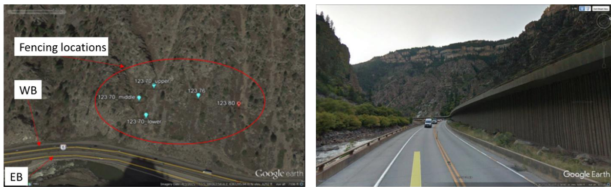
Figure 14. Site 2 near MP 123.7 in Glenwood Canyon
