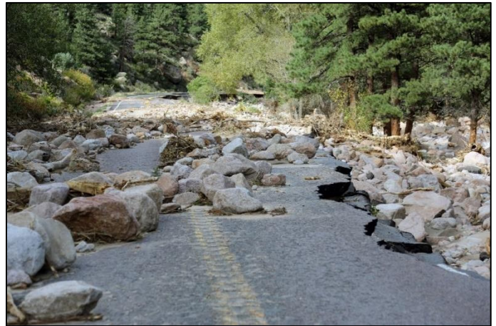
Figure 1. Flood-roadway Damage
