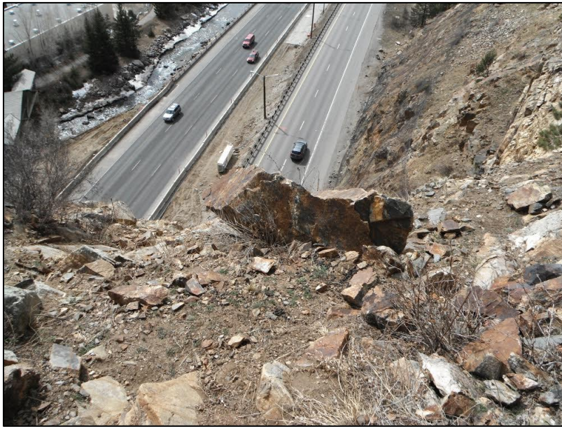
Figure 20. Rockfall Potential near Twin Tunnels on I-70
