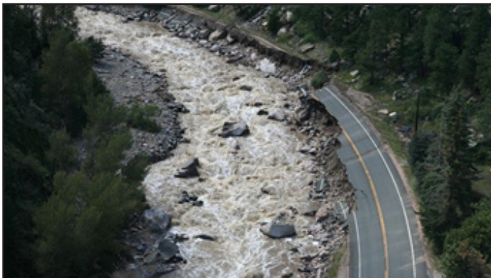
US 34 Big Thompson Canyon Flooding, 2013
