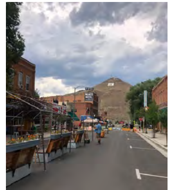
Salida, Colorado - Beginning stages of repurposing F Street to accommodate commerce amid COVID precautions.
