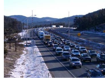
Traffic checkpoint at I-70 Floyd Hill.
