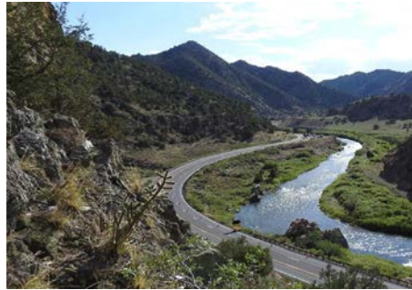
Project completed on US 50, Fremont county.
