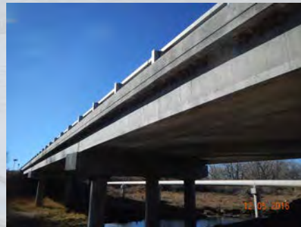
O-19-R (Purgatoire River Bridge)
