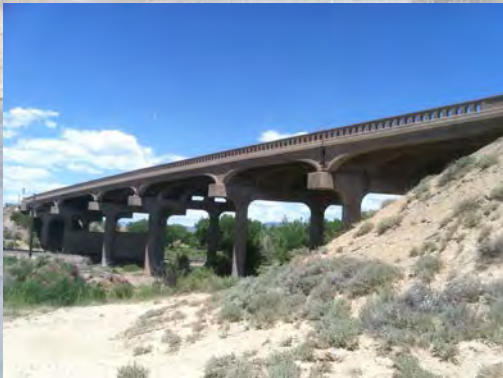
Rio Grande Railroad Viaduct, 2015
