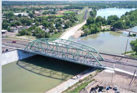
Santa Fe Avenue Bridge, Pueblo County, Rehab
