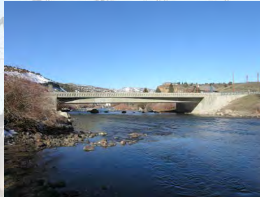
Structure F-10-AH, (Wolcott)
