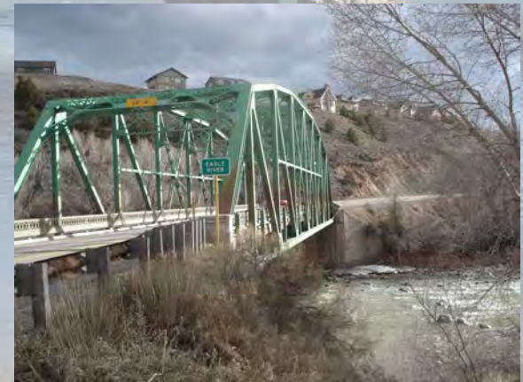
Eagle River Bridge, Eagle County, 2012
