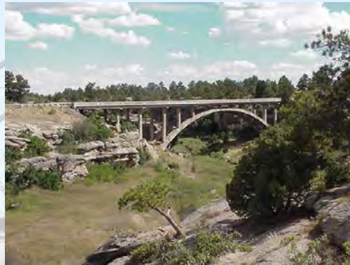
Cherry Creek Bridge, Douglas County, Rehab
