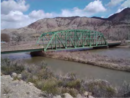
Dotsero Bridge, Eagle County, 2013
