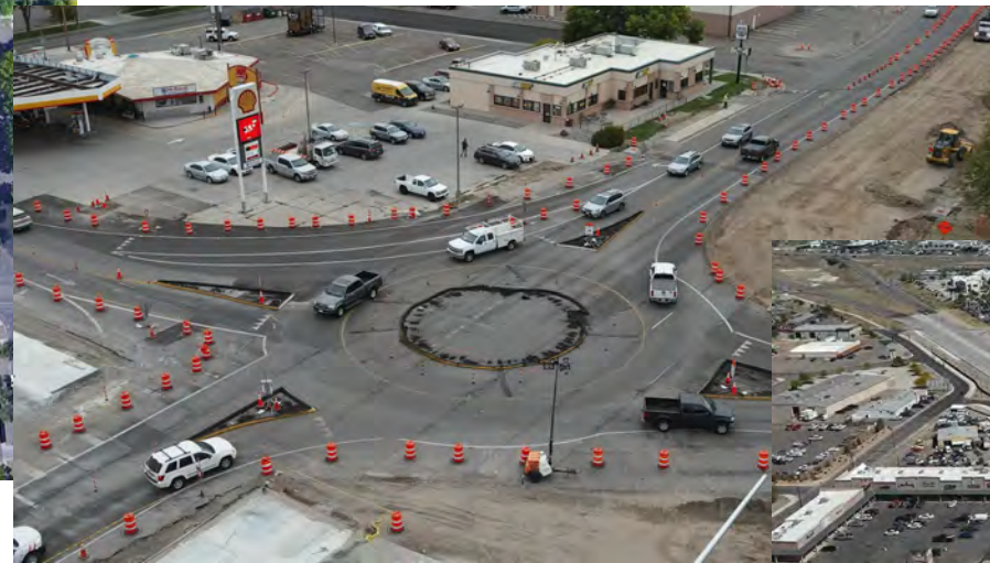
Temporary traffic circle
