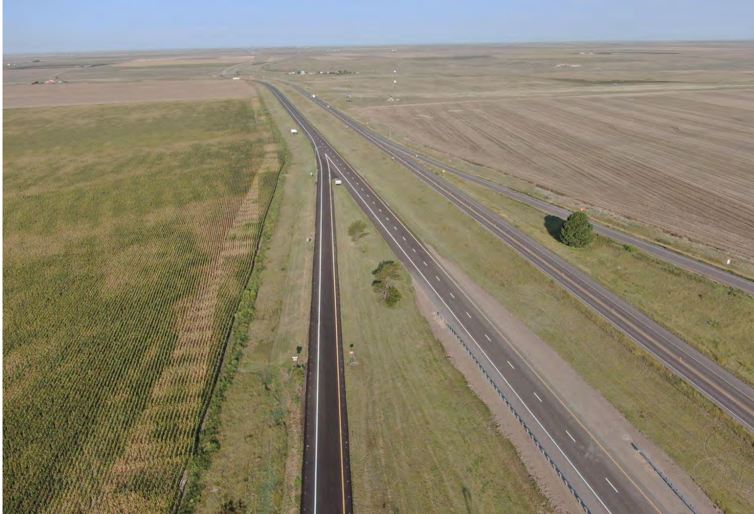
Bethune Interchange looking westbound
