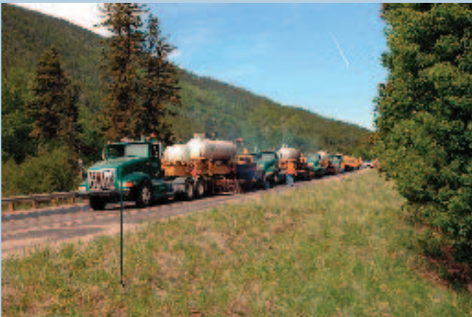
Region 1: Resurfacing US 285 on Kenosha Pass
