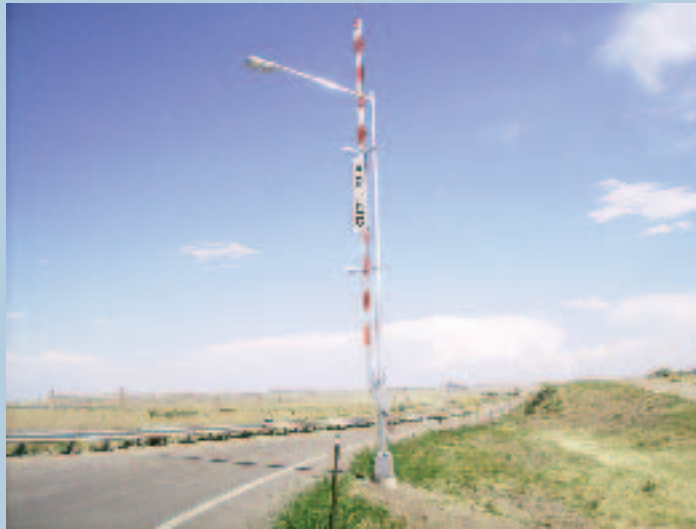
Region 2: US 24 at Garrett Road intersection improvements
