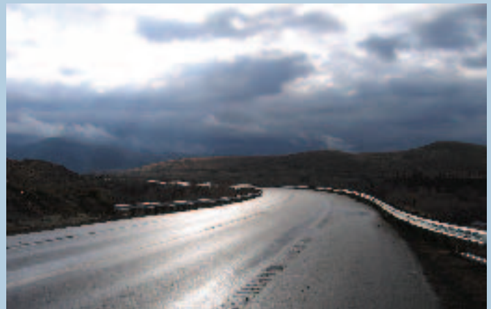
Region 3: Resurfacing US 40 east/west of Parshall
