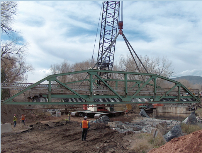
Region 4: Bridge replacement on US 34, Big Thompson Canyon
