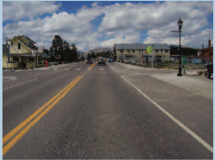
Region 1: New curb, gutter, streetlights on SH 9 through Fairplay
