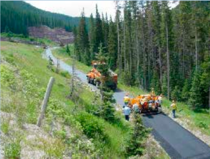
Region 1 & 3 Maintenance crews resurface the Vail Pass multi-use trail
