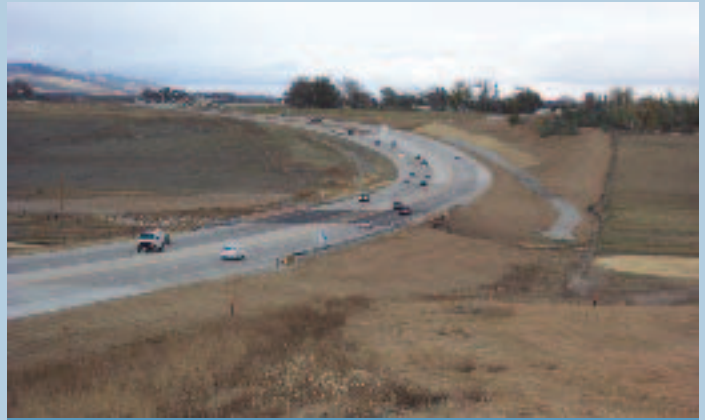
US 287 Broomfield to Loveland Corridor (Berthoud Bypass shown) Completed 2006
