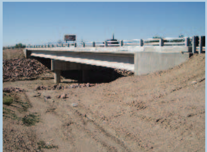
Region 2: New bridge on I-25 at Steel Hollow
