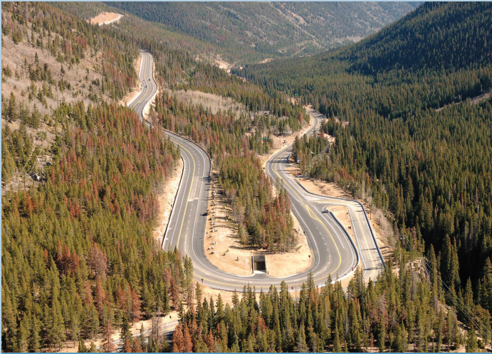
US 40 Berthoud Pass Corridor - Completed late 2006
