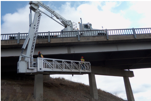
Maintenance workers conduct a routine bridge inspection on US 85 near Nunn. [REGION 4]
