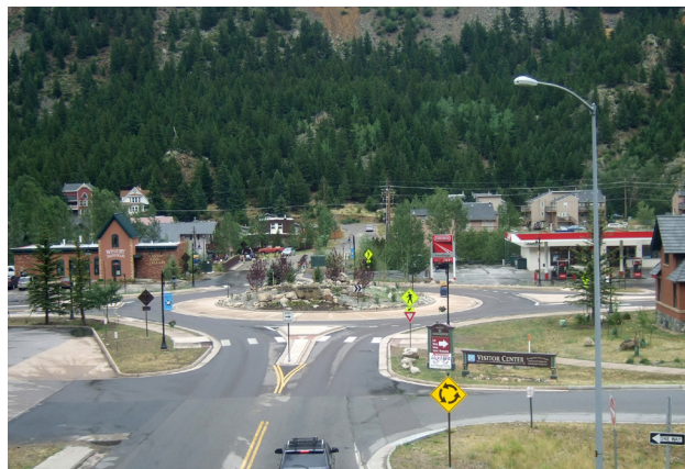
Federal funding covered a third of the $1.5 million cost of Georgetown's new roundabout. Constructed at the connector road to I-70, it provides better traffic flow and easier access for emergency vehicles responding to incidents on I-70. [REGION 1]
